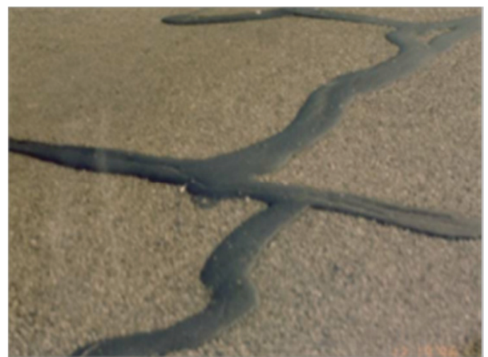
Photograph 4-3. Excessive overbanding (22).
