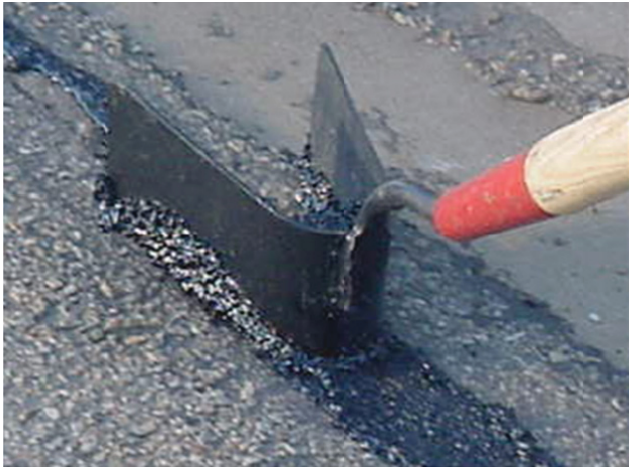
Photographs 4-1. Squeegee for sealant (hot-poured sealant on left, cold-poured sealant on right) (21).
