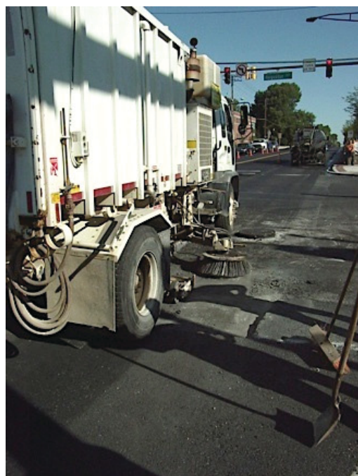
Photograph 4-6. Pavement sweeping (photo by Dale Decker).
