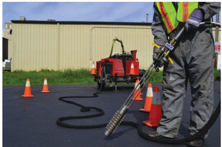
Photographs 4-9. Hot air lances (left: courtesy Crafcfo, right: courtesy Lab Mfg.).
