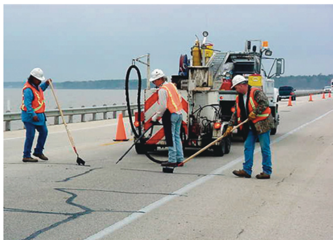
Photograph 4-15. Crack treatment operations (21).
