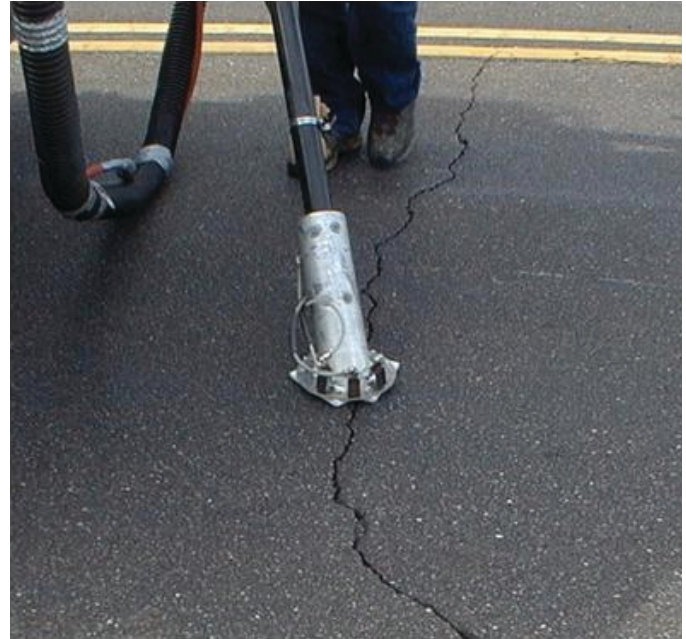
Photograph 4-8. Crack vacuum (courtesy Crafcfo).
