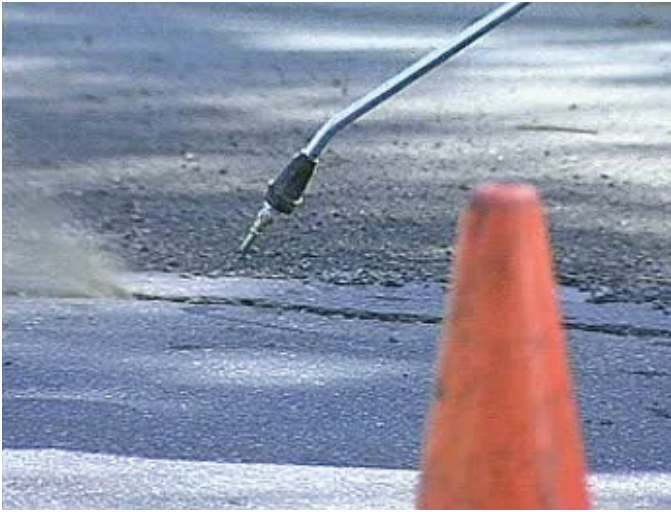
Photograph 4-7. Compressed air cleaning of crack (courtesy Crafcfo).
