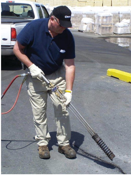
Photograph 2-4. Hot air lance (courtesy CrafcO).
