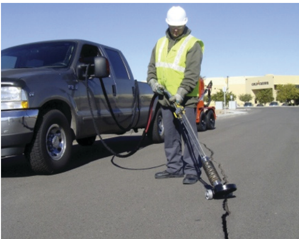
Photographs 4-9. Hot air lances (left: courtesy Crafcfo, right: courtesy Lab Mfg.).
