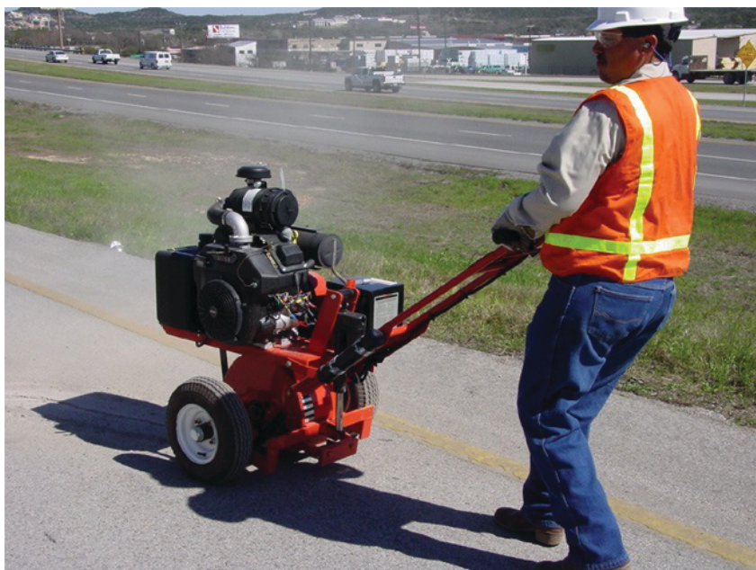
(B) Crack router (21).
