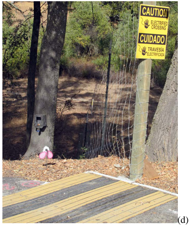
Figure 1.7. Methods used by Caltrans to avoid wildlife mortality at the transportation–wildlife interface include (a) wildlife fencing, (b) escape ramps, (c) crossing passages at culverts and bridges, and (d) electric wildlife crossing deterrent mats at unfenced intersections.
