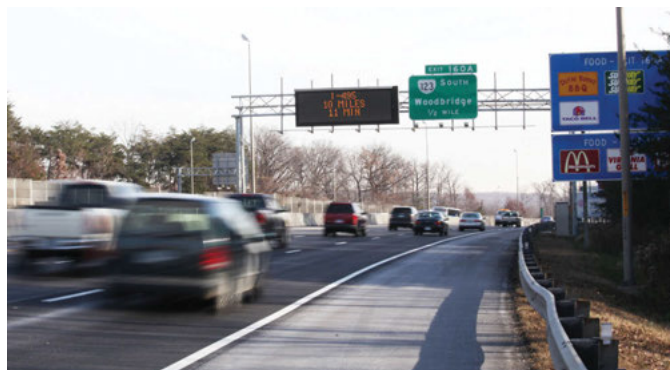
A changeable message sign on I-95 in Virginia shows travel times to an upcoming exit. Virginia and other states have robust performance management plans that address a variety of system needs.
