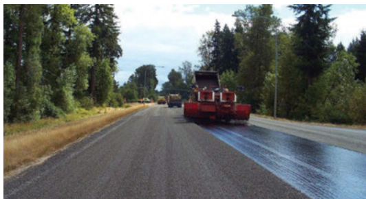
PHOTO: WASHINGTON STATE DEPARTMENT OF TRANSPORTATION
