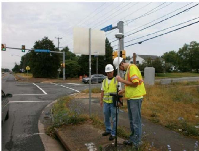
**Figure 3.93.** Establishment of survey control before geophysical investigations during in-service testing.
