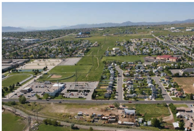
Figure 46. Urban and suburban portion of the project before construction (Credit: UDOT).
