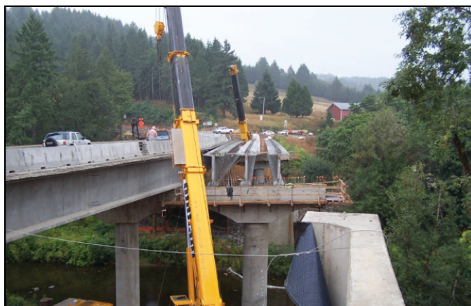
Figure 11. Bridge 01601 under construction (Credit: OBDP).
