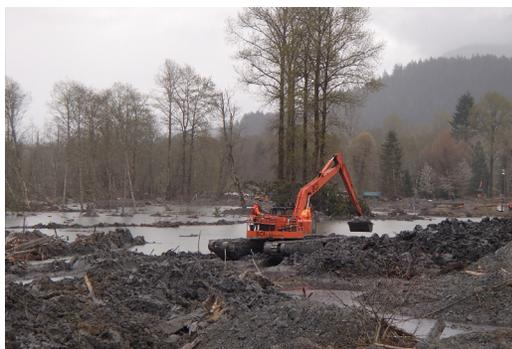
Amphibious excavator constructing a pilot channel to increase flow through the debris dam after the March 22, 2014, landslide—the deadliest in U.S. history—near Oso in northwestern Washington State.
