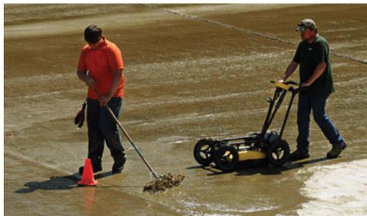
Contractors use a ground-penetrating radar device on the Gavins Point Dam spillway in South Dakota.
