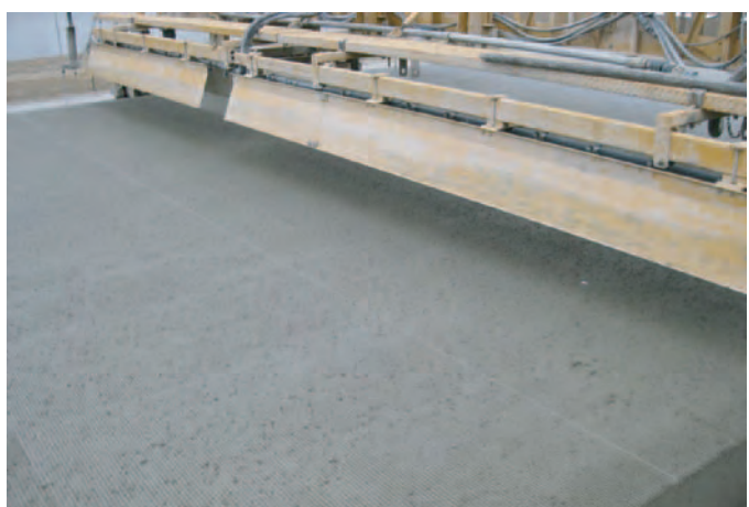
Figure A.8. Transverse tining.
