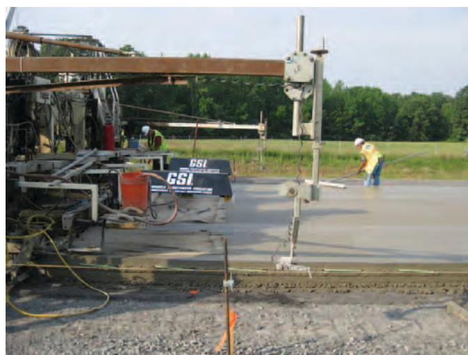
Figure 2.46. Paver-mounted GSI setup.
