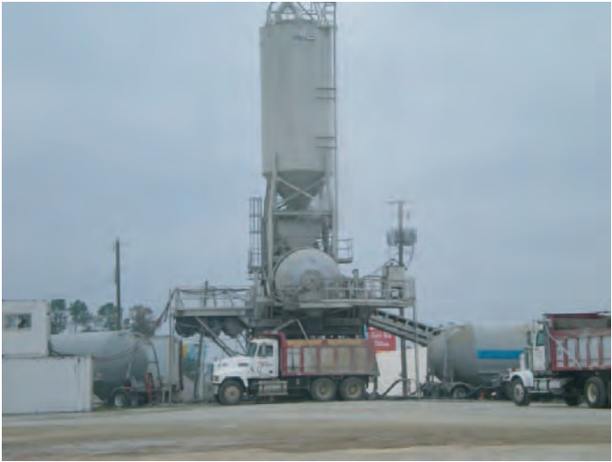
Figure A.2. Central mix batch plant used for paving I-75 Northbound.
