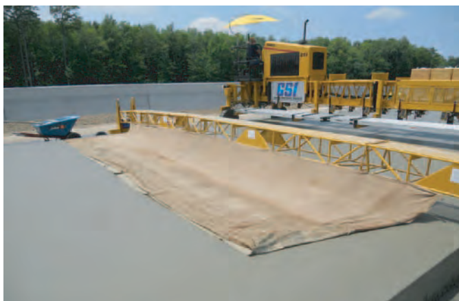
Figure A.7. Burlap drag behind hand finishers.
