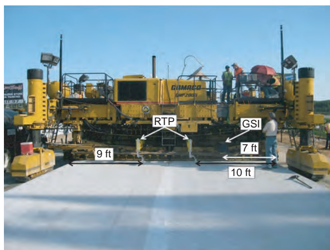
Figure 2.14. Day 1 (May 10) paver-mounted real-time profilers' setup.
