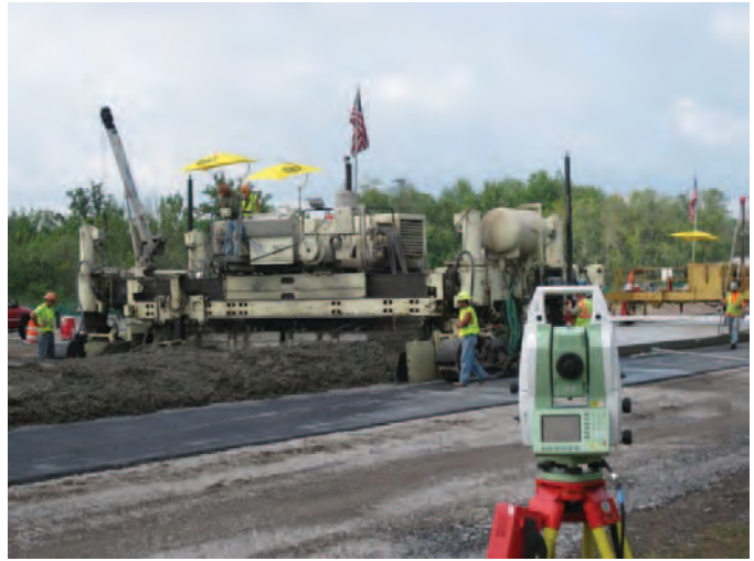
Figure 2.68. Stringless guidance system used on New York paving project.
