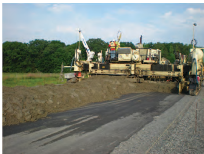
Figure 2.40. Guntert & Zimmerman 850 slipform paver.
