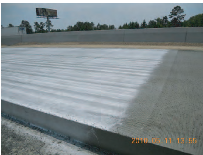
Figure A.9. Curing compound applied.
