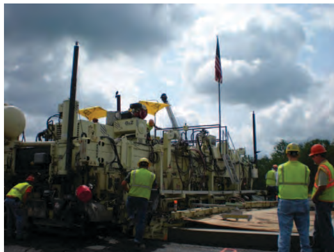
Figure 2.66. Guntert & Zimmerman 850 slipform paver.
