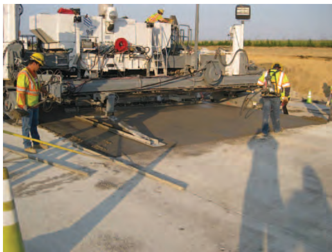
Figure 2.50. Guntert & Zimmerman 850 slipform paver and final finisher.
