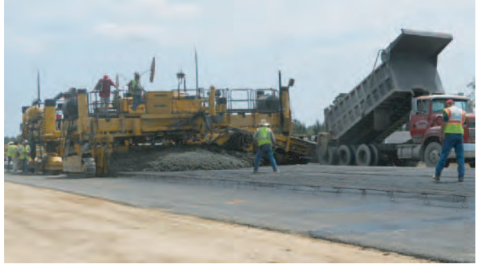
Figure A.3. Front view of GOMACO PS 2600 belt placer/spreader.
