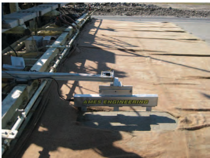
Figure 2.70. Location of Inertia-Link sensor on paver-mounted Ames Engineering RTP without dowels.
