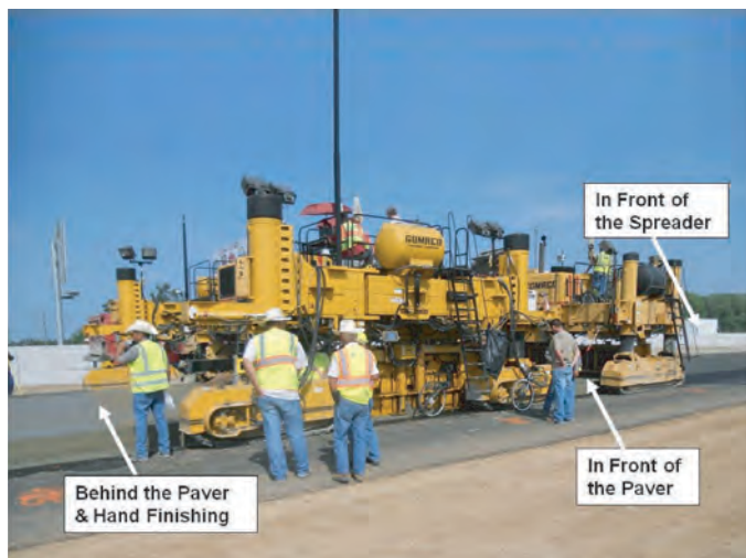
Figure 2.9. Rear view of paving train and note-taking stations.
