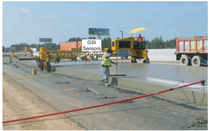
Figure 2.16. GOMACO GSI machine setup behind hand finishers.
