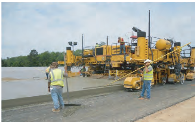
Figure 2.13. Note-taking station: behind the paver.
