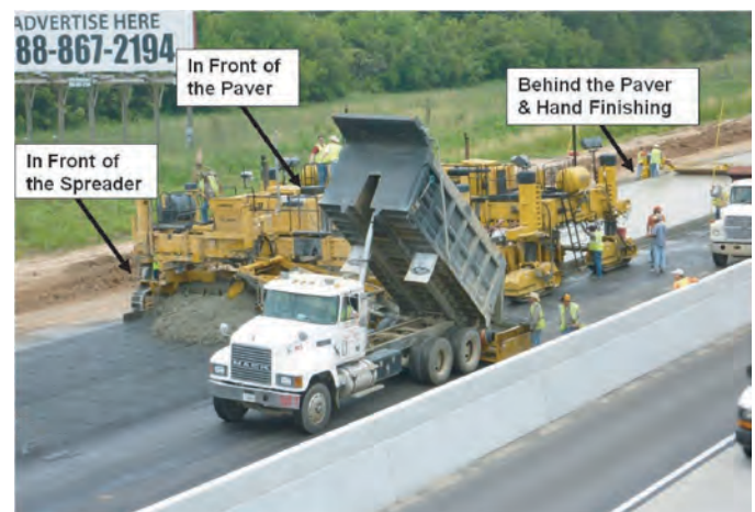
Figure 2.8. Front view of paving train and note-taking stations.
