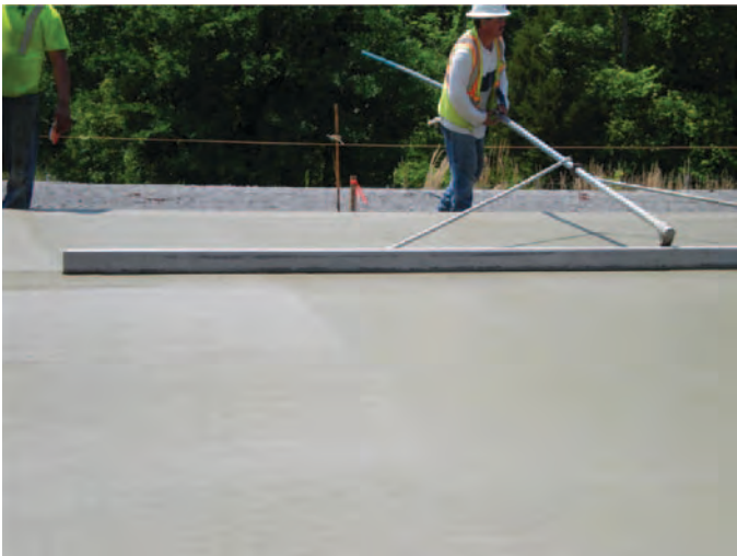
Figure 2.41. Straightedge used to identify bumps and dips.
