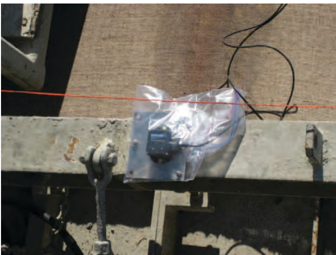
Figure 2.54. Inertia-Link mounted to the beam fixed to the finishing pan.
