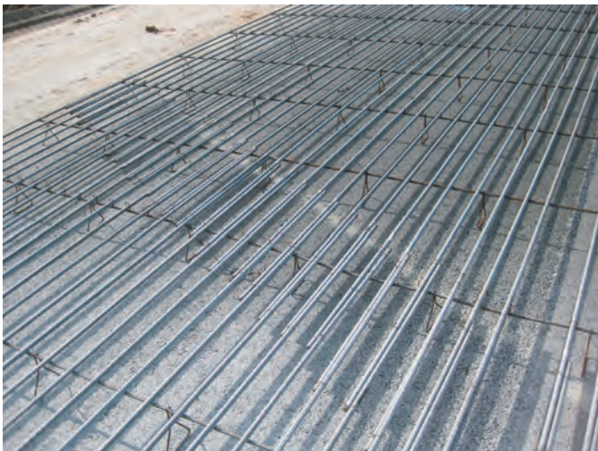
Figure 2.32. Reinforcement in place before placement of the concrete.
