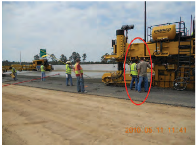
Figure 4.1. Paving superintendent interacting with the GSI display on the side of the paver.
