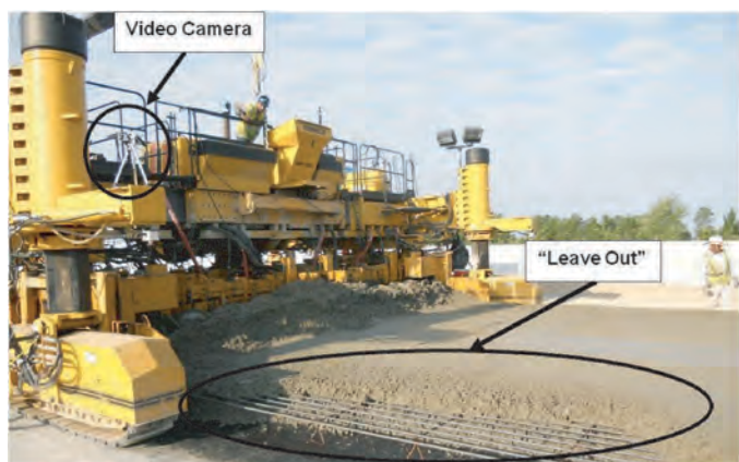
Figure 2.12. Note-taking station: in front of the paver.
