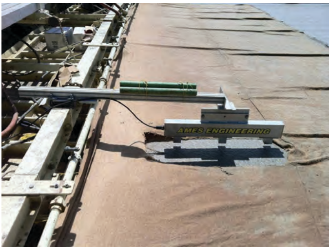
Figure 2.64. Contractor-owned RTP equipment mounted to the rear of the paver.
