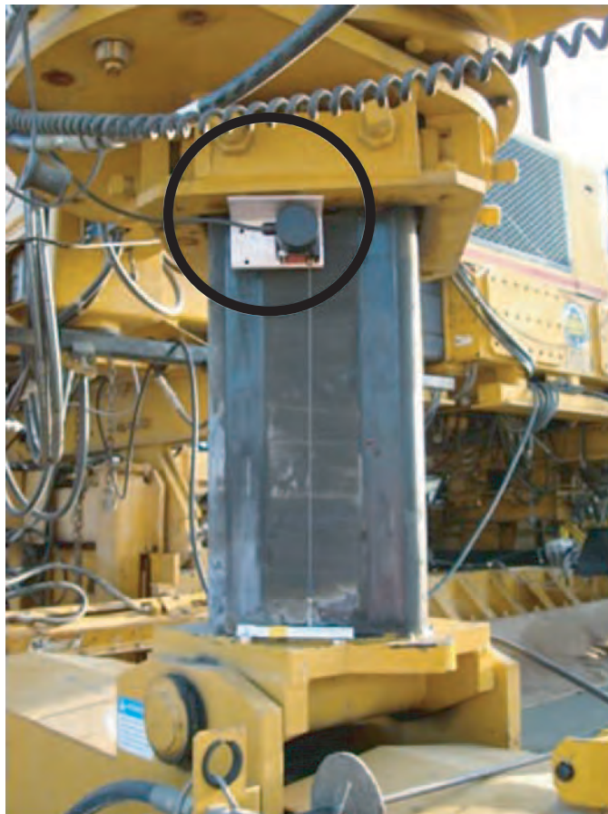
Figure 2.20. Draw wire sensor mounted on leg of paver.
