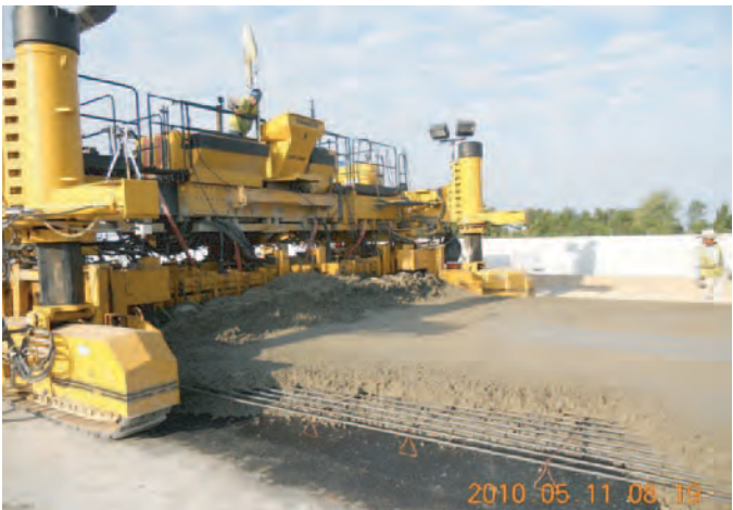
Figure A.4. Front view of GOMACO GHP 2800 slipform paver.
