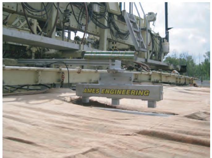
Figure 2.3. Ames Engineering RTP mounted behind a paver.
