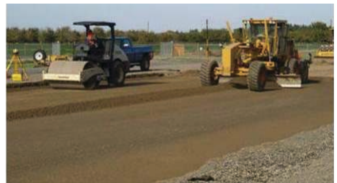
Figure 2.24. Compaction and grading of test track aggregate base.
