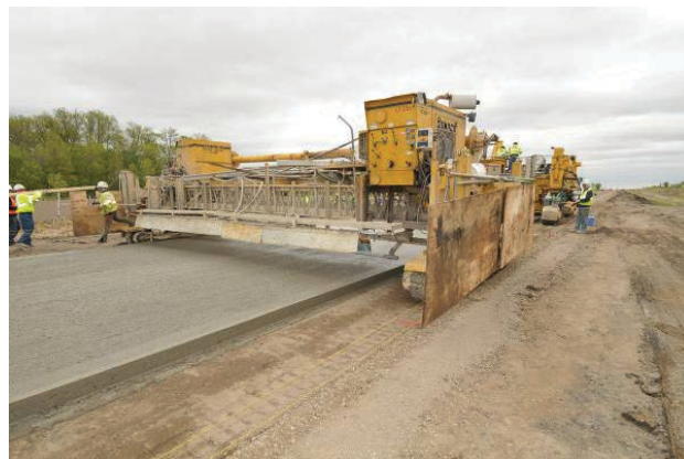
Figure 2.18. Tining the PCC surface to provide texture for mechanical bonding between PCC and HMA layers.
