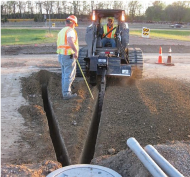
Figure 2.11. Installing conduits to carry and protect the instrumentation cables.
