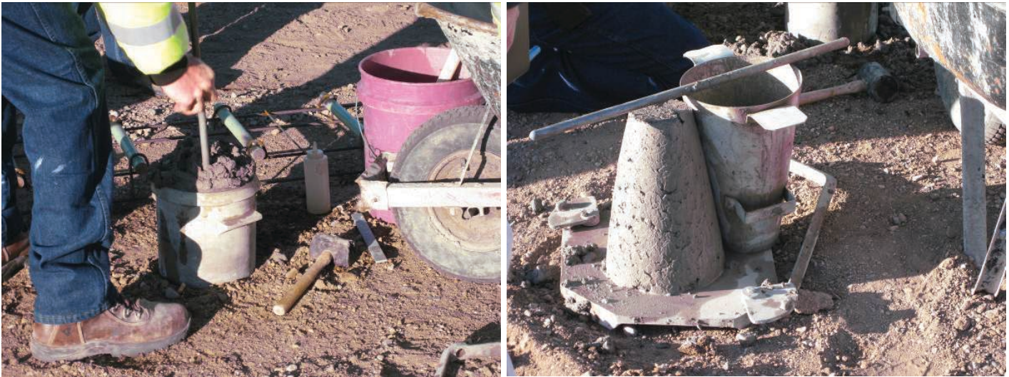
Figure 5.3. QA testing of the PCC layer for entrained air and slump.
