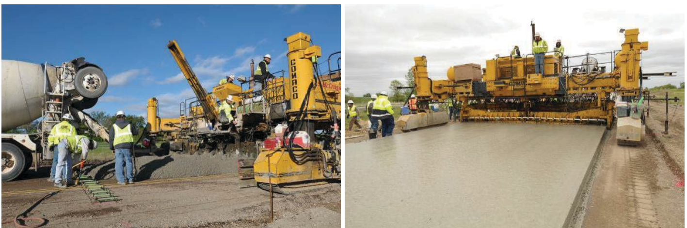
Figure 5.2. Paving the PCC layer.
