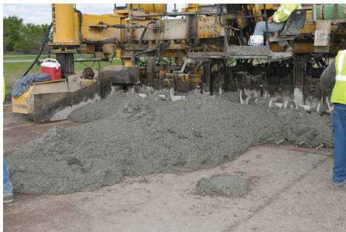
Figure 2.16. Placement of PCC layer on the aggregate base.
