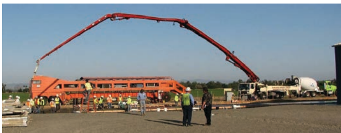
Figure 2.30. View from east, concrete pump.
