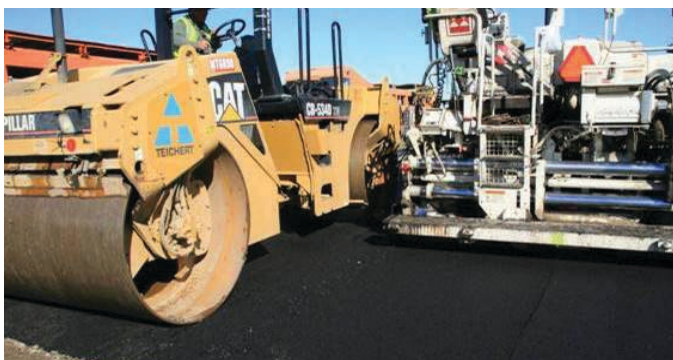
Figure 2.34. Compaction and placement of RHMA-G in Lanes C and D.
