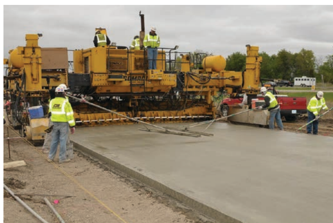
Figure 2.17. Finishing the PCC surface to remove surface irregularities.
