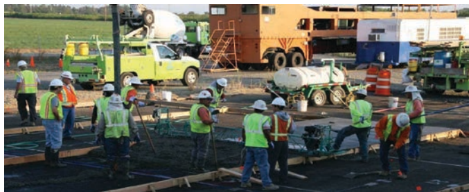
Figure 2.32. Motorized screed on Lane C, Day 1 PCC paving.
