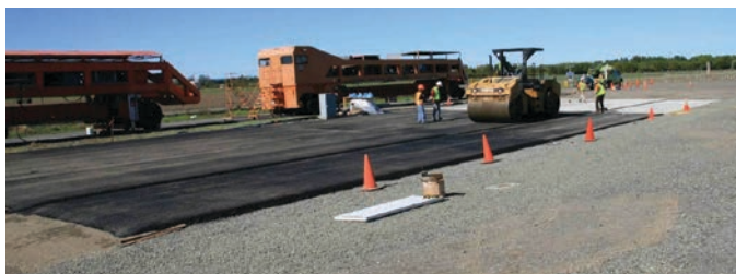
Figure 2.36. Completed test track showing two HMA lift thicknesses and PCC sections.
