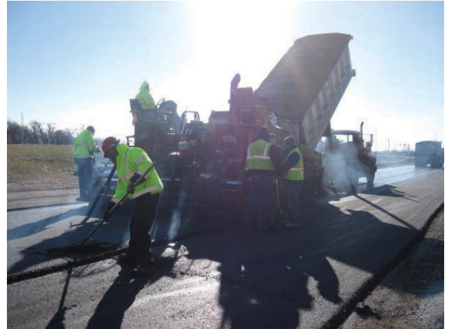
Figure 2.41. Placement of HMA lift onto lower PCC layer.
