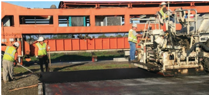
Figure 2.33. Start of PG64-28PM placement following application of tack coat.
