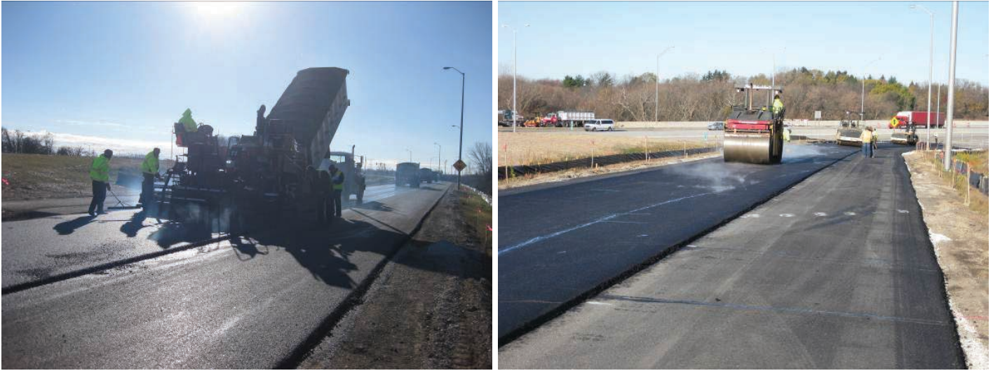
Figure 5.7. Placing and compacting HMA layer for HMA/PCC composite pavements.
