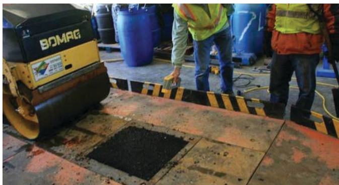
Figure 2.37. Compaction of ingots with rolling wheel compactor.
