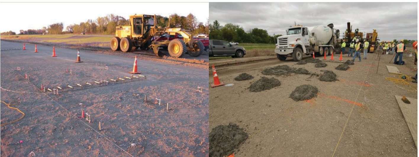
Figure 2.15. Overview of instrumentation packed in concrete before PCC paving.
