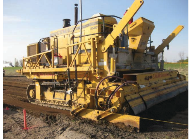
Figure 2.9. Trimming the subgrade using a string line and trimmer.
