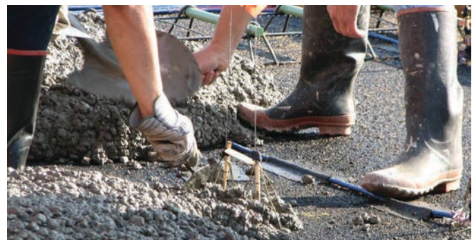
Figure 2.31. Hand packing concrete around instrumentation.
