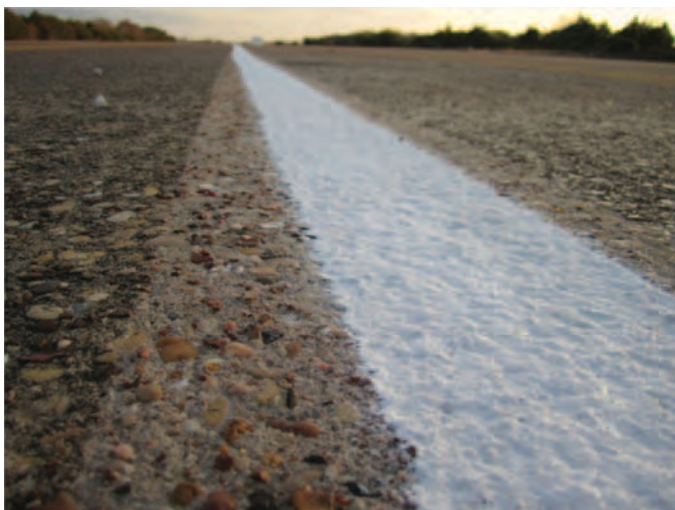
Figure 55. Installed markings on cleaned concrete.
