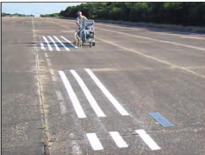
Placing two 20-foot stripes for each of the 5 bead packages. Measuring retroreflectivity after 24 hours.
