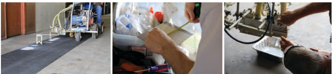
Figure 49. Calibrating the Graco striping equipment.
