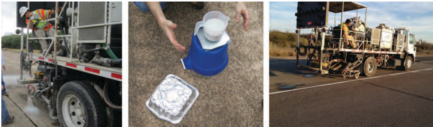
Figure 54. Calibrating the full-sized long line paint striper.
