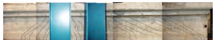
Figure 34. Flexural failure observed in Test BT.8.Typ.2.
