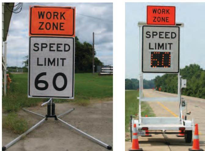
**Figure 13. Examples of some technologies to implement short-term speed limits in work zones.**
