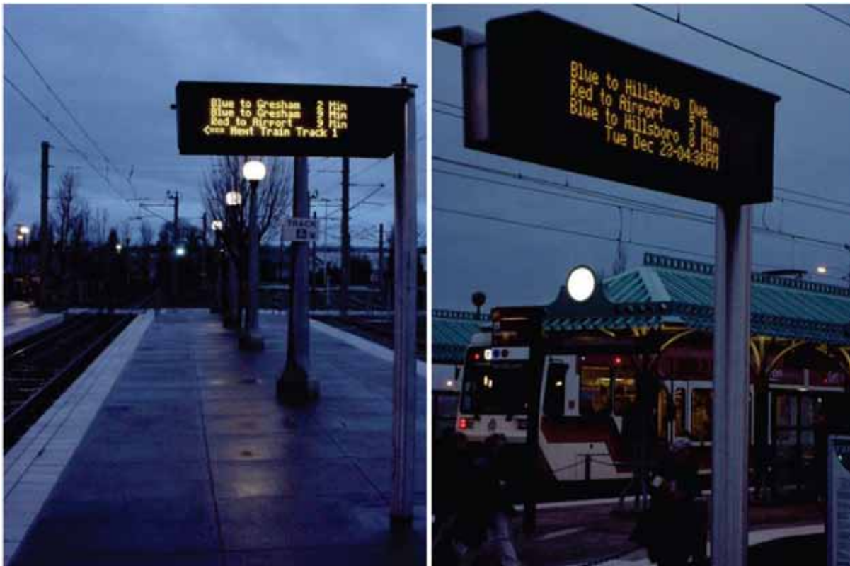
FIGURE 52 DMS on light rail platform (Courtesy: TriMet).
