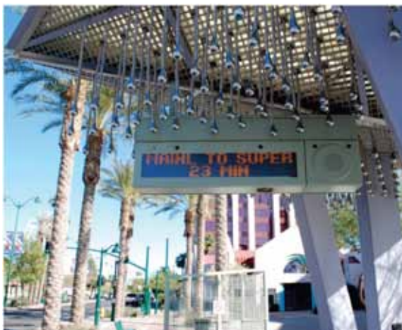
FIGURE 24 Mesa (Arizona) BRT station DMS (Courtesy: TranSystems 2011).
