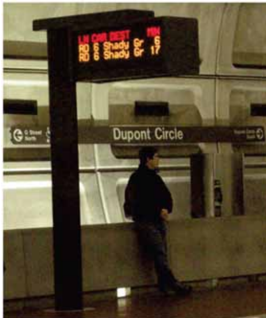
FIGURE 23 WMATA DMS in Dupont Circle Metrorail Station (Courtesy: Carol Schweiger 2007).
