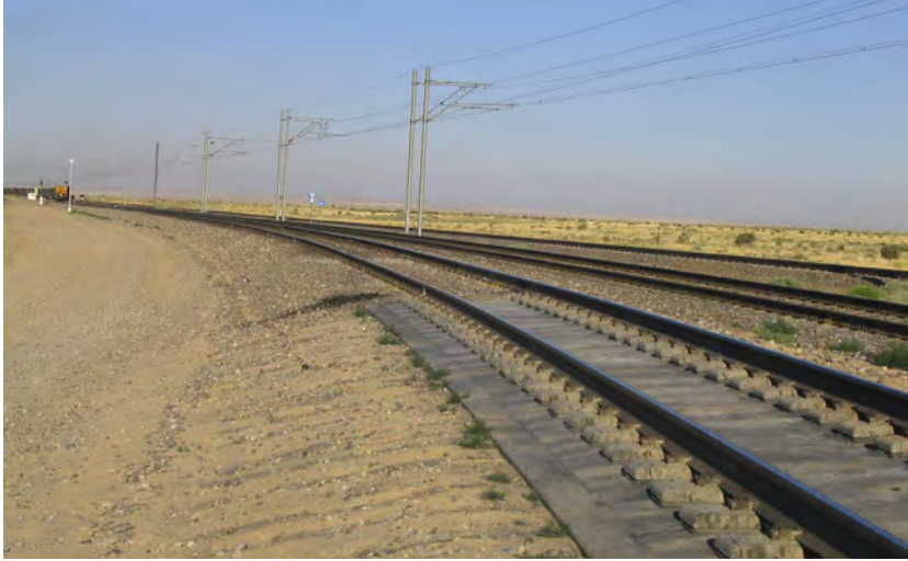
Transition from slab track to ballasted track at demonstration test, Transportation Technology Center, Inc.
