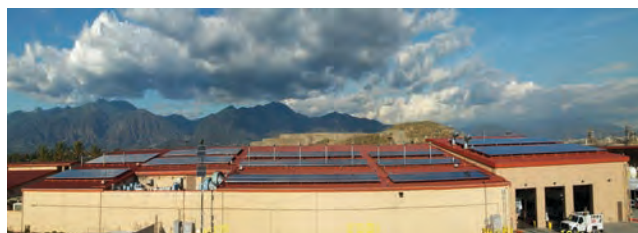
FIGURE 18 Solar panels on a foothill transit maintenance facility. Courtesy: Foothill Transit.
