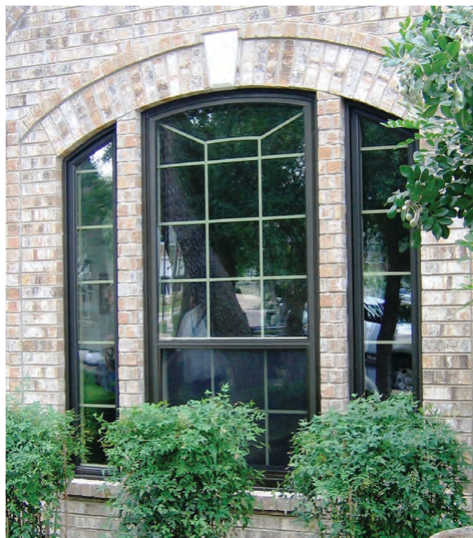
Figure 9.2. Acoustical replacement window.
