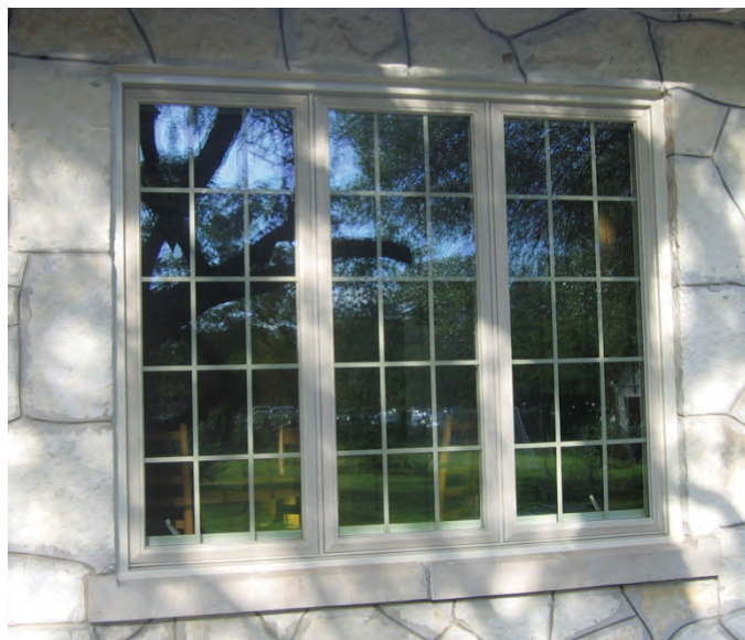
Figure 9.8. Acoustical casement unit.
