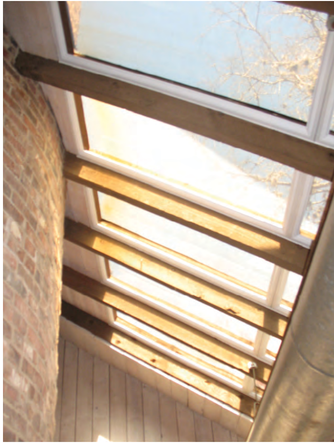
Figure 9.12. Secondary skylight system.
