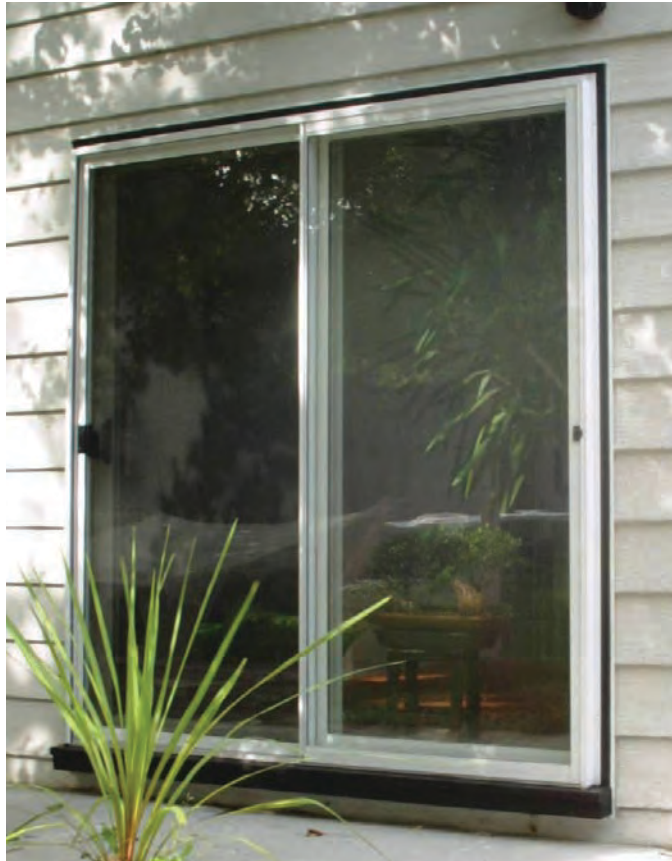
Figure 9.14. Secondary sliding patio door.
