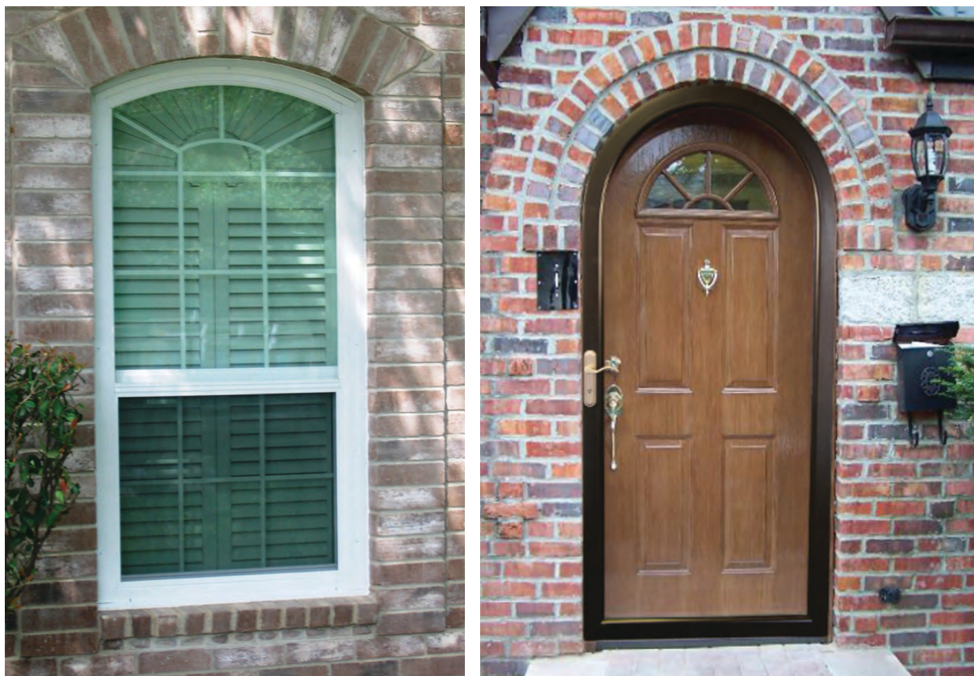
Figure 9.13. Secondary window and secondary storm door.
