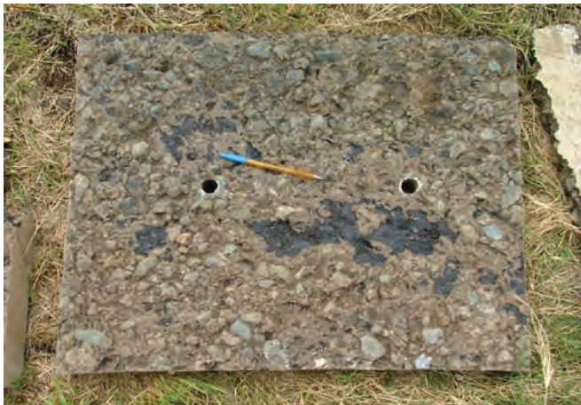
a) Investigation of slab underside
