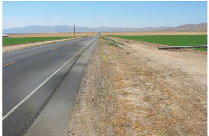
Figure 4.5. Irrigation water sprays on the road.
