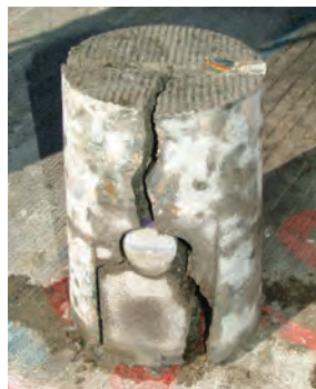
Failure around dowel bar on pre-cast slab
