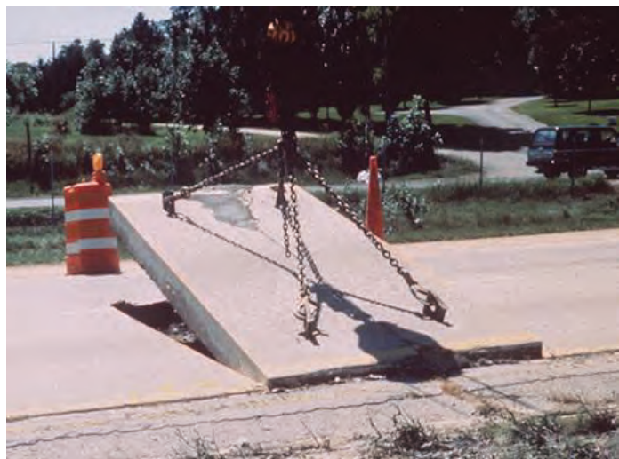
Figure 7.13. Removing and checking PCC slabs.
