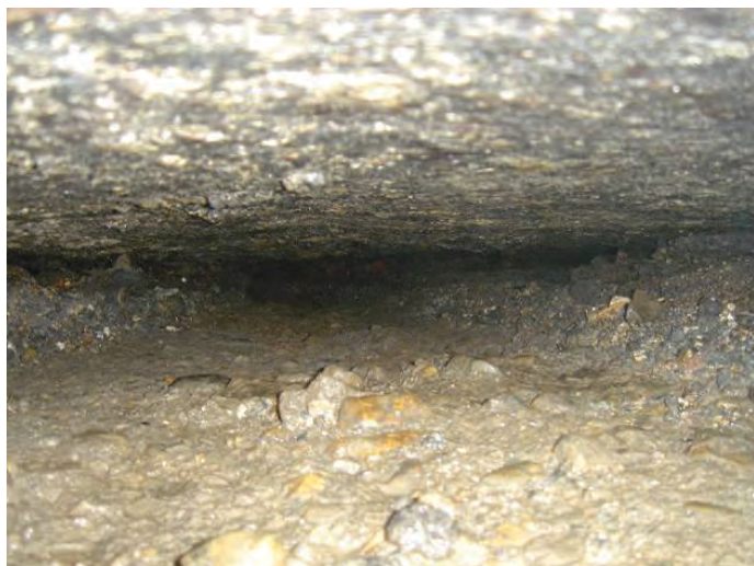
Figure 7.6. Borescope views of void under concrete pavement.
