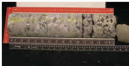
Assessment of tie bar location (middle of PCC) and permeable cement treated base (right side of core)
