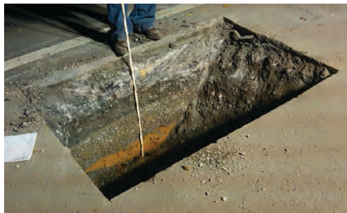
(Photo courtesy of Virginia Department of Transportation)
