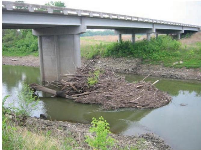
**Figure 1.1.** *Drift accumulation on a single bridge pier (photo courtesy of Ayres Associates).*
