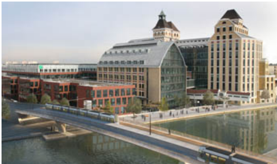
FIGURE 9 Paris T3 Line extension: new bridges and adjacent urban development.
