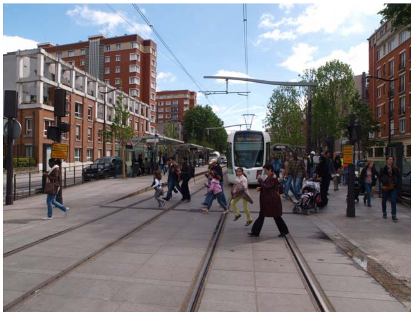
FIGURE 3 Typical LRT stop. Modern stops are integrated with their surroundings, creating a public realm that allows easy pedestrian accessibility and promotes TOD (Paris, France).
