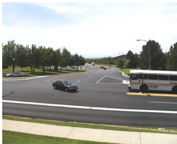
FIGURE 5 South Campus Drive–Campus Center Drive intersection before the roundabout construction. Yield signs control the traffic along the top of the T-intersection. Bypass lanes existed at the two corners and across the top of the T. Because of the existing free movements the change to a roundabout operation was not as extreme for drivers.
