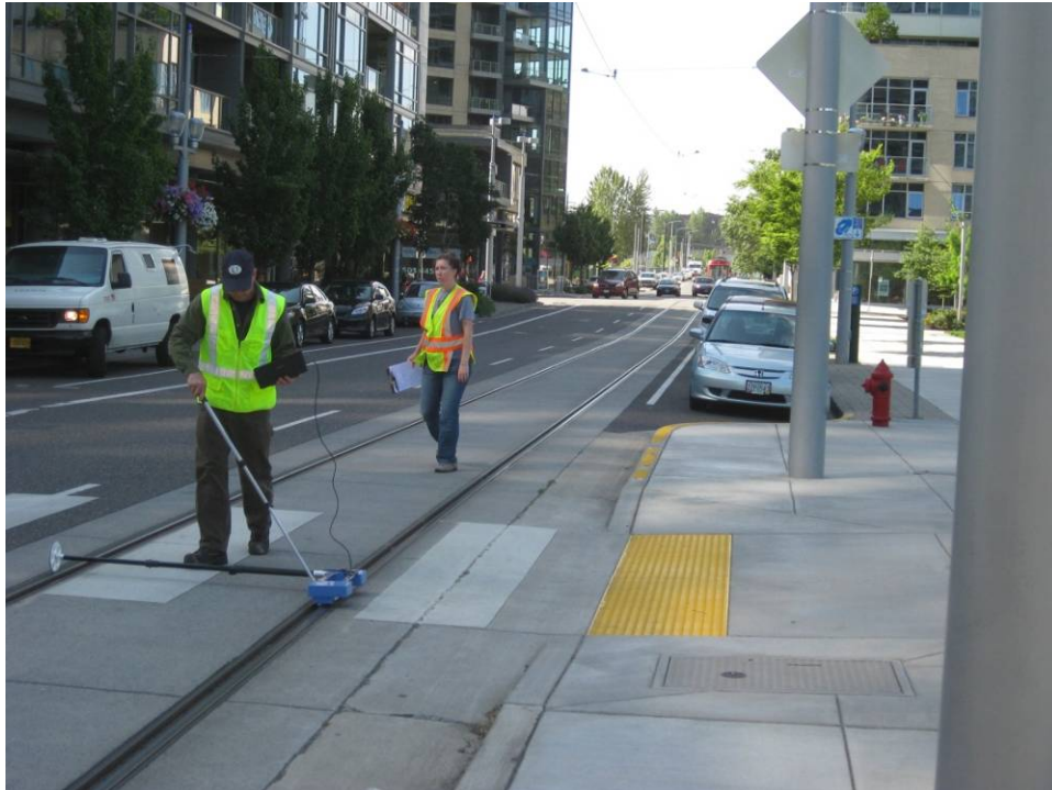
FIGURE 11 Rail roughness measurement in Portland streetcar tracks (12).
