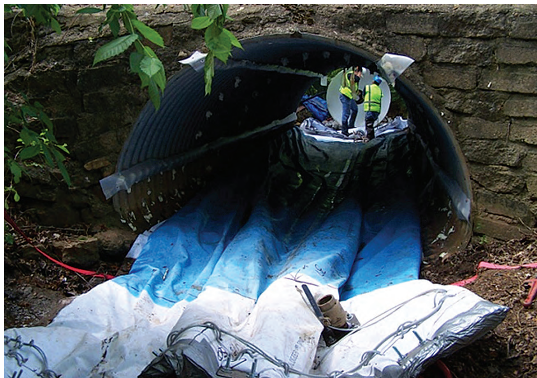
Conventional CIPP liner inserted into host pipe.
