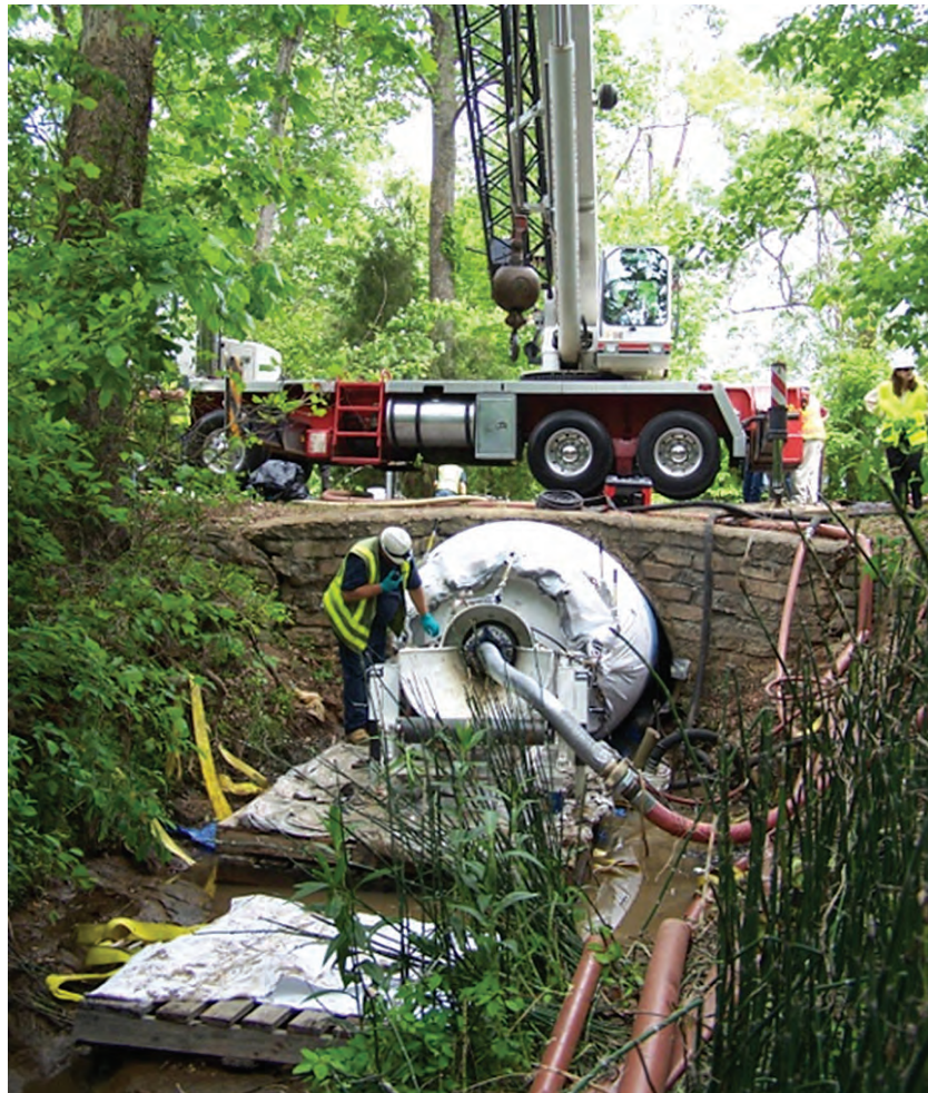
Conventional CIPP steaming process.
