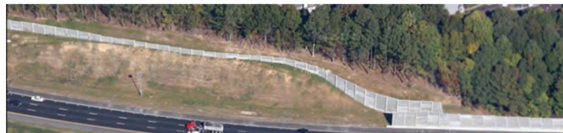
Bird's-eye view of I-40–Jones Franklin Road noise wall.
