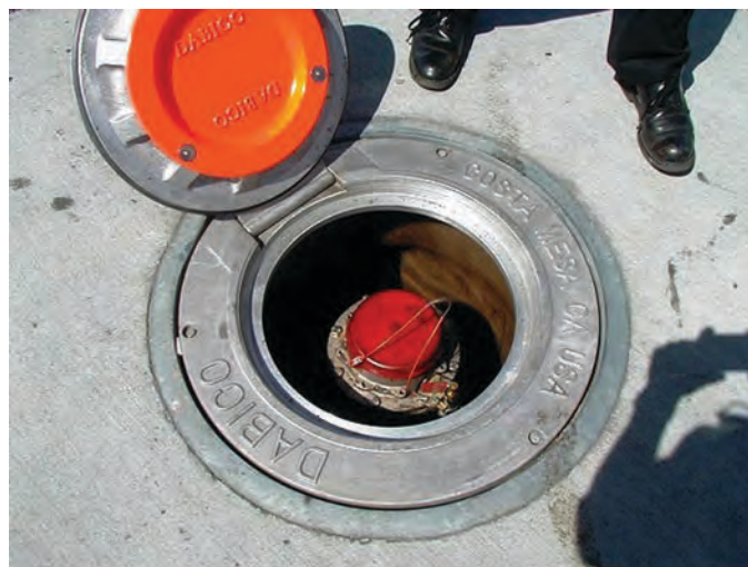
Figure 4-38. Hydrant fuel pit.
