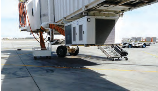
Figure 3-27. Bridge-mounted preconditioned air unit.
