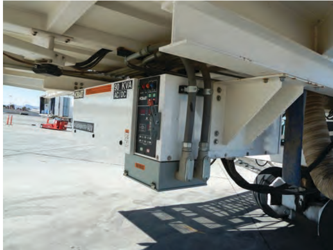
Figure 3-31. Bridge-mounted ground power unit.
