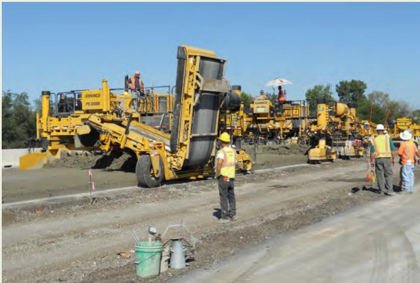
A two-lane belt paver spreads the top lift of concrete over a bottom lift of “green” concrete in front of a slip-form paver, creating a composite pavement on the Reagan Memorial Tollway.
