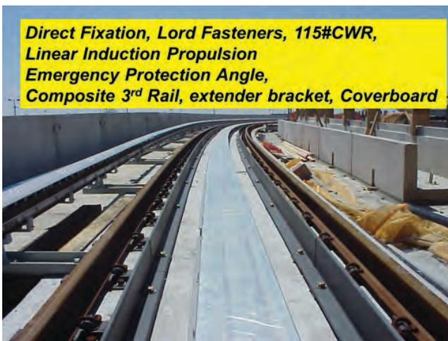
FIGURE 8 Direct fixation (DF) track.
