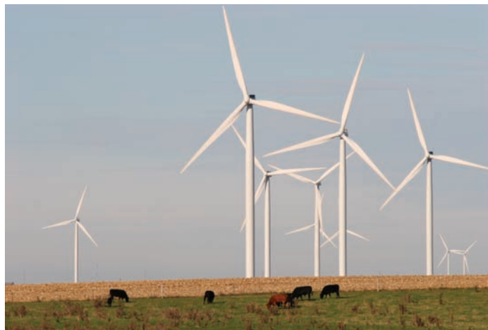
FIGURE 3.6 Wind farm. SOURCE: http://www.dis.anl.gov/projects/windpowerforecasting.html . Used with permission from U.S. DOE's Office of Science.
