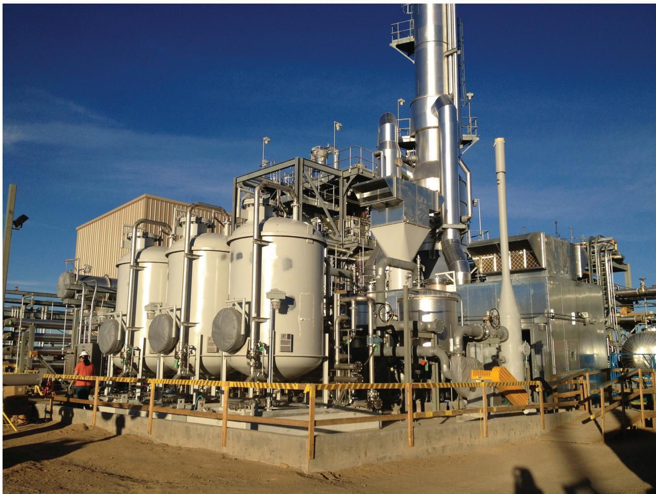
FIGURE 3-2 Brine reduction system installation at PCAPP. NOTE: The three tanks in the center-left foreground are granular activated carbon adsorbers for the product distillate. SOURCE: Provided courtesy of PCAPP staff.
