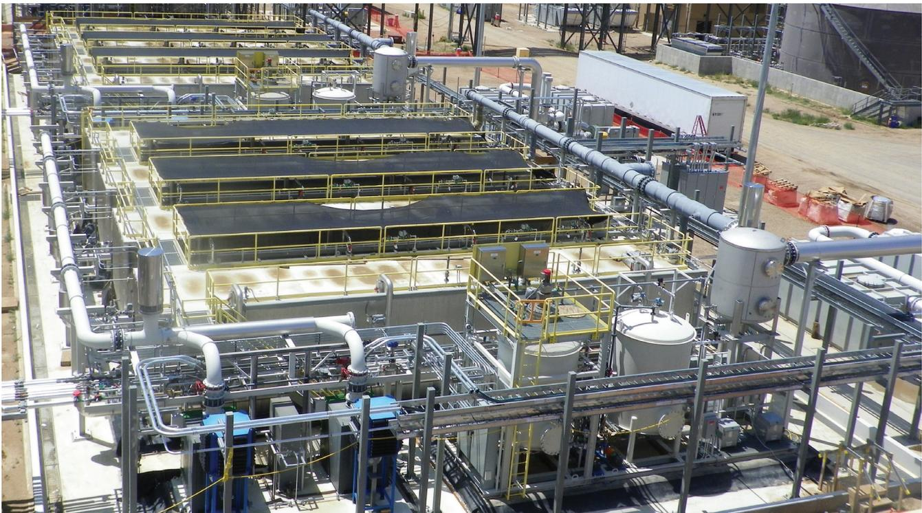
FIGURE 2-2 Two of the four biotreatment modules at PCAPP, each of which has four immobilized cell bioreactor units. SOURCE: Paul Usinowicz, Water/Wastewater Research Leader, Battelle, “Design and Operating Conditions for PCAPP’s Biotreatment Process,” presentation to the committee, November 28, 2012.
