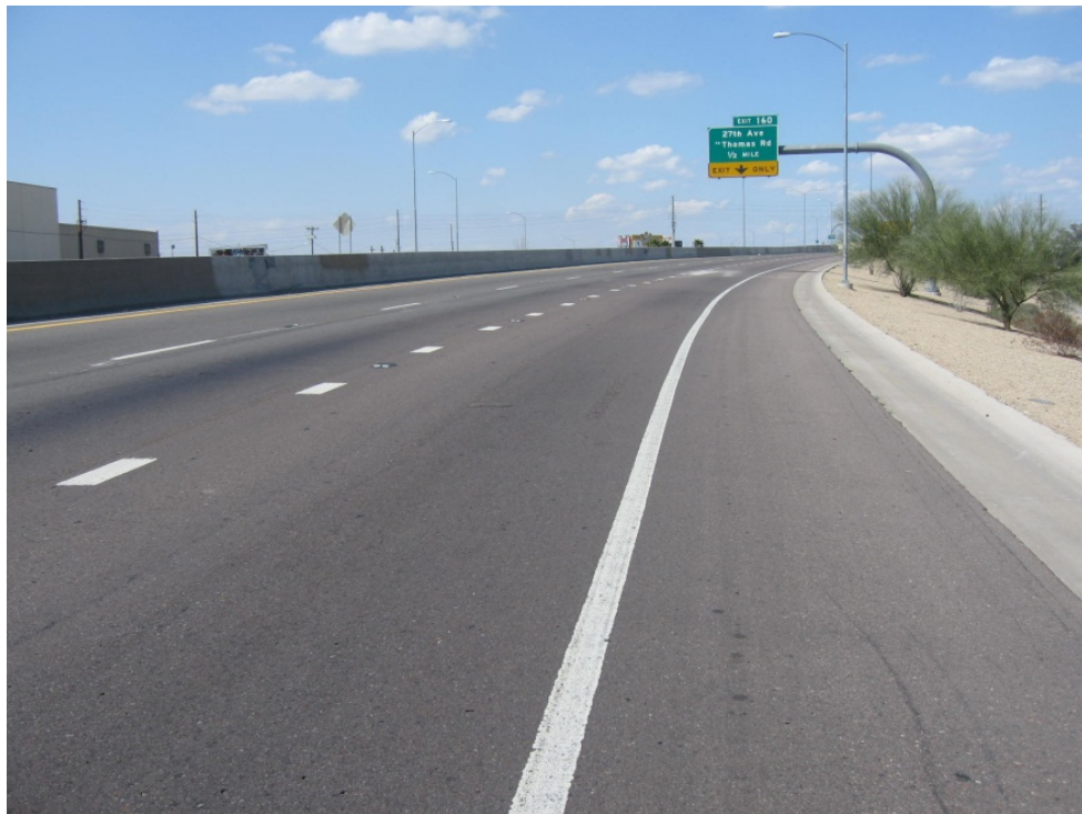
FIGURE 10 Intersection of US-60, Thomas Road, and 27th Avenue in Phoenix, March 2010.
