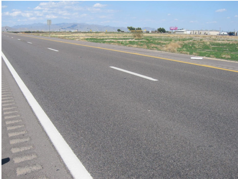
FIGURE 9 US-85 near Buckeye, Arizona, March 2010
