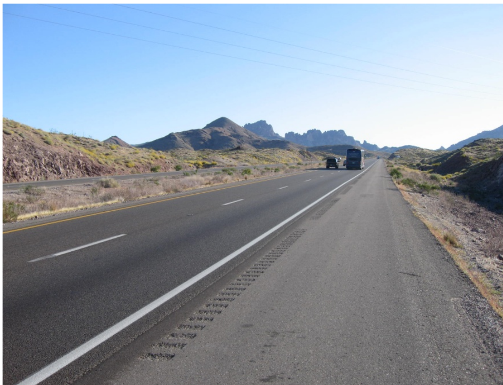
FIGURE 5 SR-68 near Bullhead City, Arizona, March 2010.
