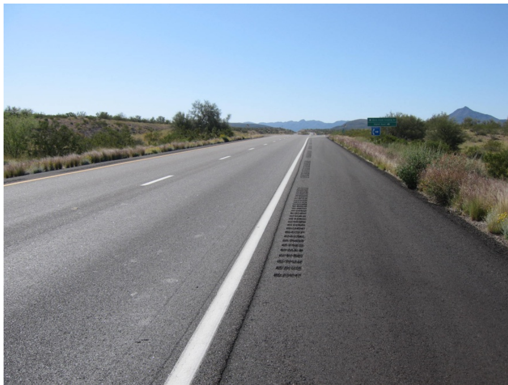
FIGURE 7 US-90 South of Wikieup, Arizona, March 2010.
