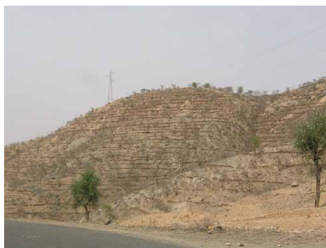
FIGURE 43 Constructed terraces on exposed slopes, Asmara-Assab Road, Eritrea (Courtesy: A. Faiz).
