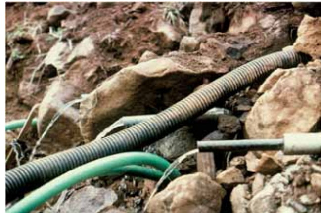
FIGURE 13 Outlet of horizontal subsurface slope drainage (Courtesy: M. Long) .
