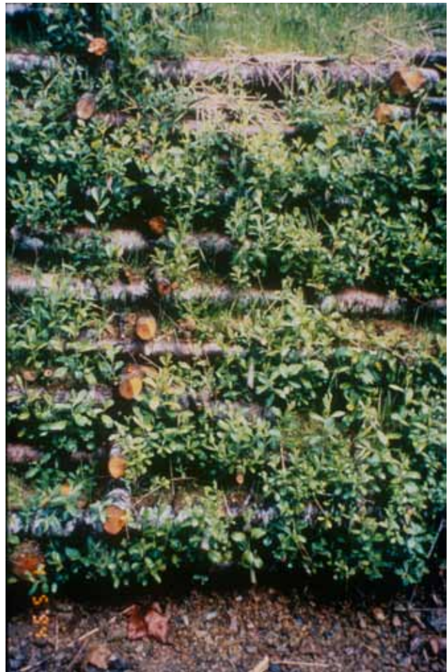
FIGURE 28 Live crib wall, from a distance (left) and close up (right) (Courtesy: G. Keller).
