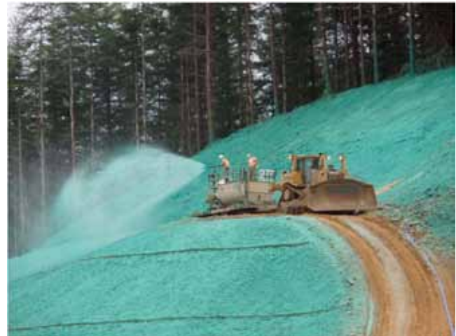
FIGURE 15 Hydro seeding of a slope (Courtesy: M. Long).
