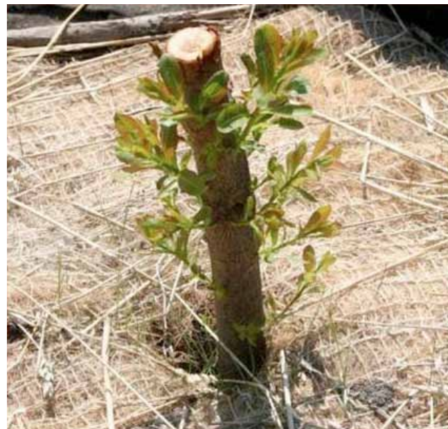
FIGURE 23 Live stake used to pin down matting (Courtesy: R. Sotir).
