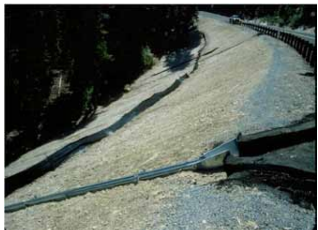
FIGURE 7 Down-drain (Courtesy: G. Keller).
