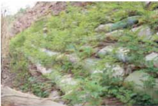
FIGURE 31 Vegetated soft gabion wall (Shah 2008).
