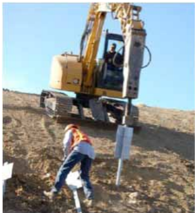
FIGURE 41 Six-foot plate piles (left) and plate pile installation (right) using an excavator with a hydraulic hammer (Courtesy: Y. Prashar).
