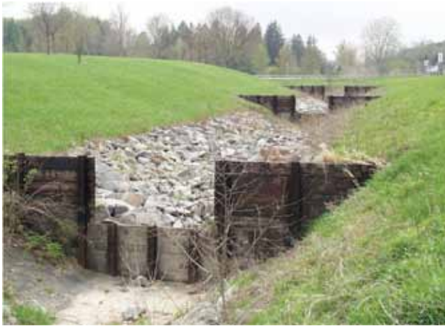
FIGURE 19 Wooden check dams with rock reinforcement (Courtesy: D. Orr).
