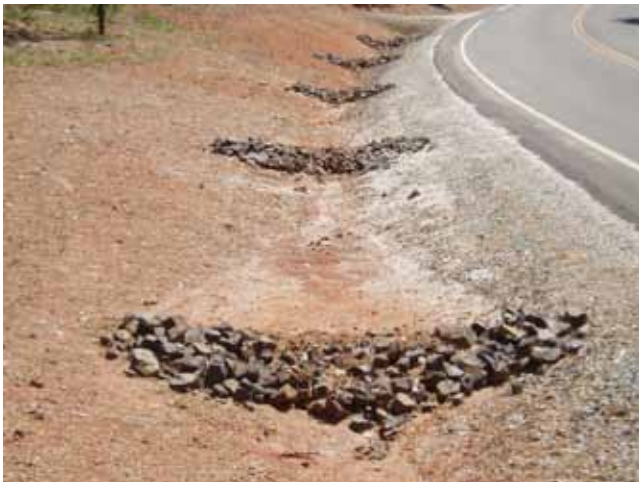
FIGURE 21 Rock pile check dams (Courtesy: G. Keller).
