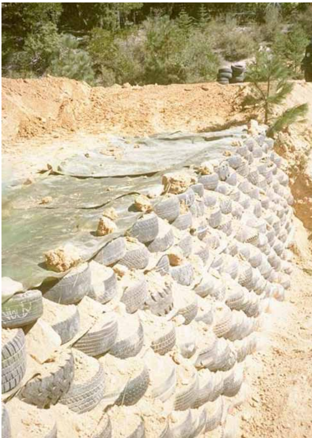
FIGURE 39 Tire wall and construction (Courtesy: G. Keller).
