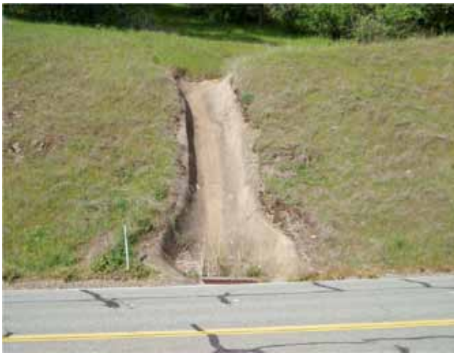
FIGURE 8 Concrete surface drainage (Courtesy: G. Keller).
