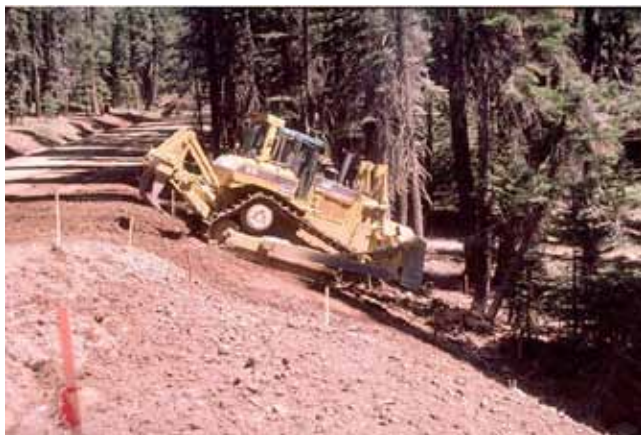
FIGURE 44 Roughened soil and trackwalking with heavy equipment (Courtesy: G. Keller).
