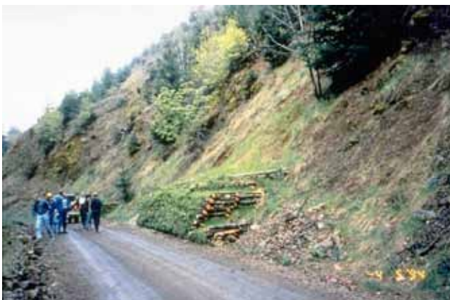
FIGURE 28 Live crib wall, from a distance (left) and close up (right) (Courtesy: G. Keller).
