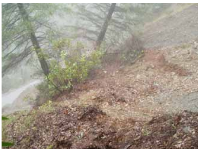
FIGURE 5 Slumped slope with leaning trees (Courtesy: G. Keller).
