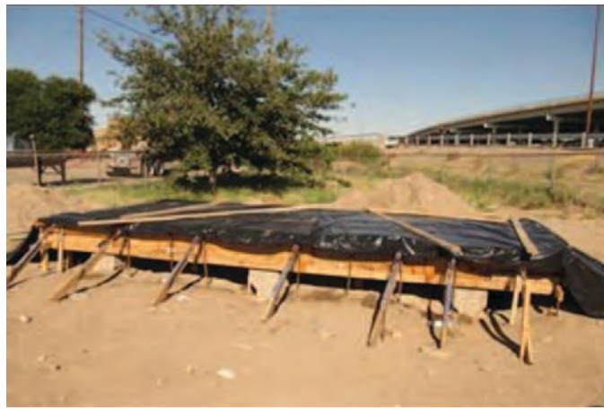
Figure 5.14. Fabricated slab: (a) schematic and (b) curing.
