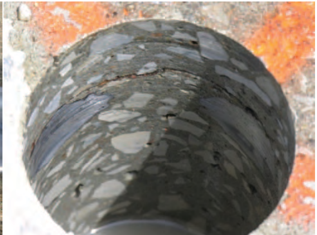
Figure 2.3. Corroded rebar in an excavated deck (top) and extracted core (bottom left), and delamination in a drill hole in a deck (bottom right).
