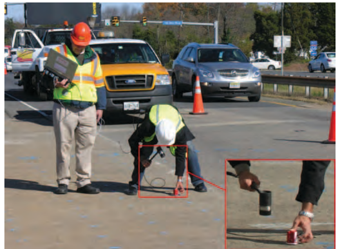
Figure 3.8. Impulse response testing.
