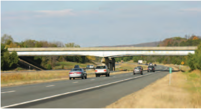
Figure 5.1. Side view of Route 15 bridge over I-66 in Haymarket, Virginia.
