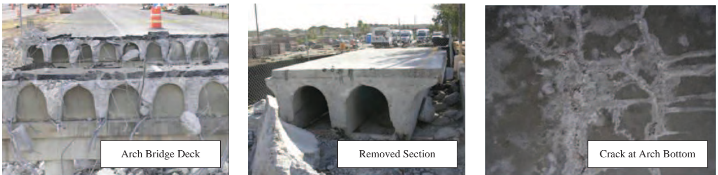
Figure 5.19. Bridge with arch deck.
