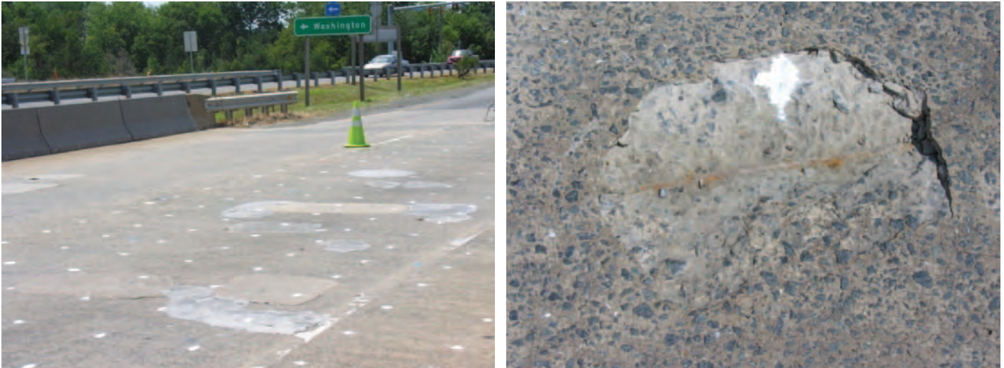
Figure 2.1. Deck deterioration.
