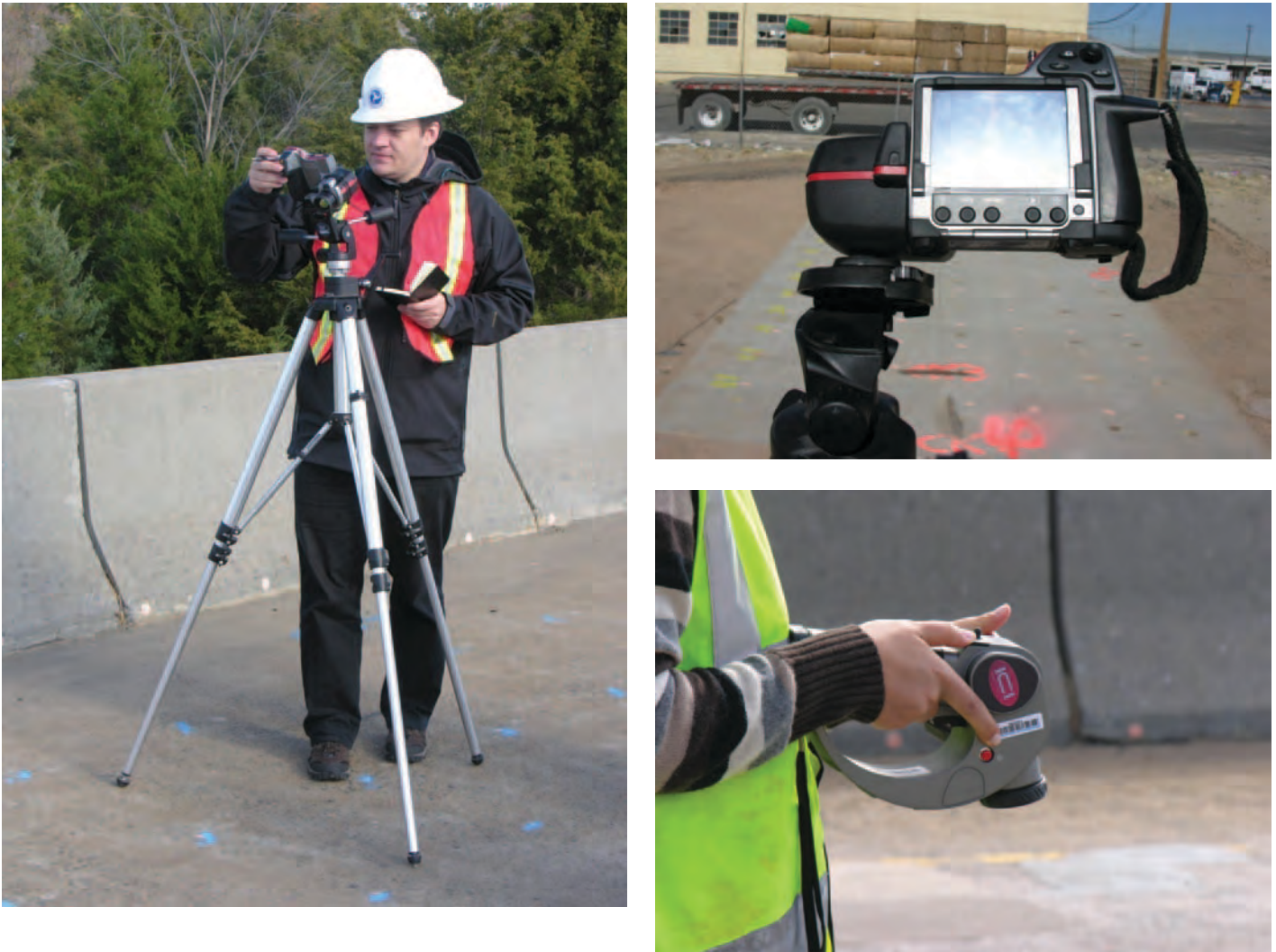
Figure 3.18. Infrared thermography testing.
