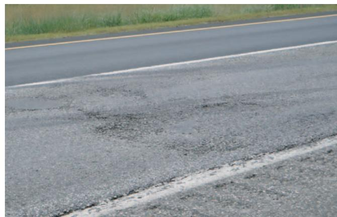
**Figure 3.69.** Damage from segregation in old HMA mat on I-295.
