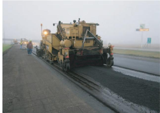
**Figure 3.54. Paving operation during Region 3 demonstration.**
