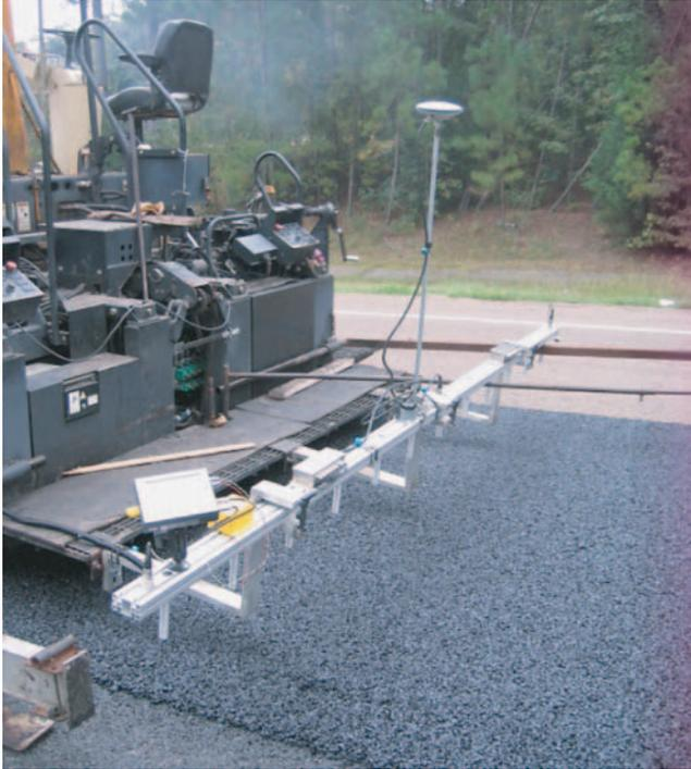
Figure 3.35. Pave-IR collecting thermal profile data on Region 4 demonstration.
