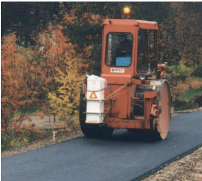
**Figure 3.17. Testing the use of GPR in HMA compaction guidance in Finland.**
