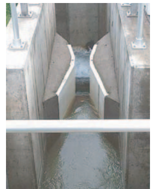
Figure 4.6. Example of a Parshall flume.
