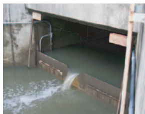
Figure 4.7. Example of a weir.
