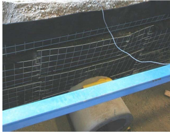
Figure C.15. Grid with Geosynthetic used for the end-wall treatment for all burial testing (shown here with 4ft of cover soil over the 24 in diameter specimen).
