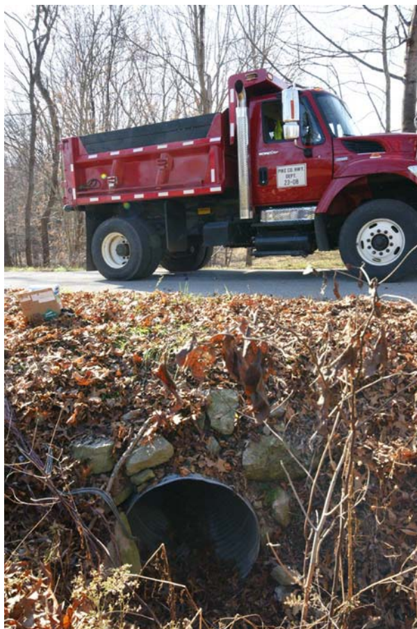
Figure D.2 Testing of CMP-D3-F2.5 under static truck loading
