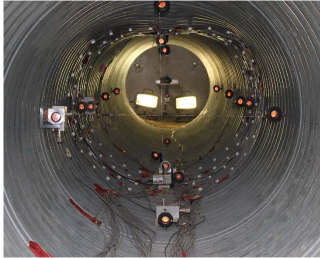
(a) Internal view
