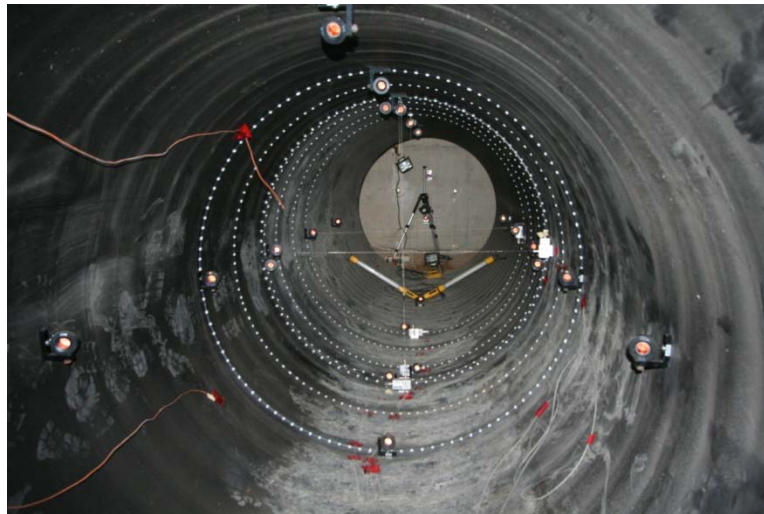
(c) Instrumented pipe
