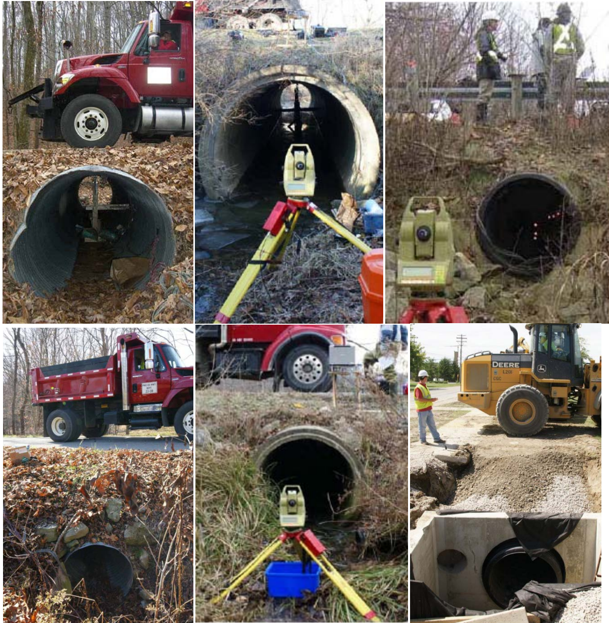
Top left (first CSP), Top Middle (first RCP), Top right (first HDPE pipe) Bottom left (second CSP) Middle (second RCP), Bottom Right (second HDPE pipe). Figure 1 Images of the six culverts in Ohio tested under vehicle loads.
