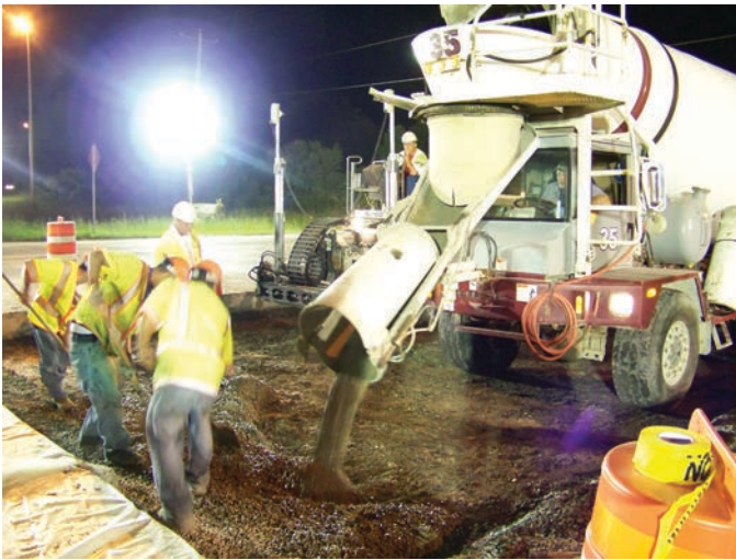
Figure 11.2. Material being directly deposited in PPCP work areas: (left) CTPB placement during Delaware project and (right) LCB placement during California I-680 project.
