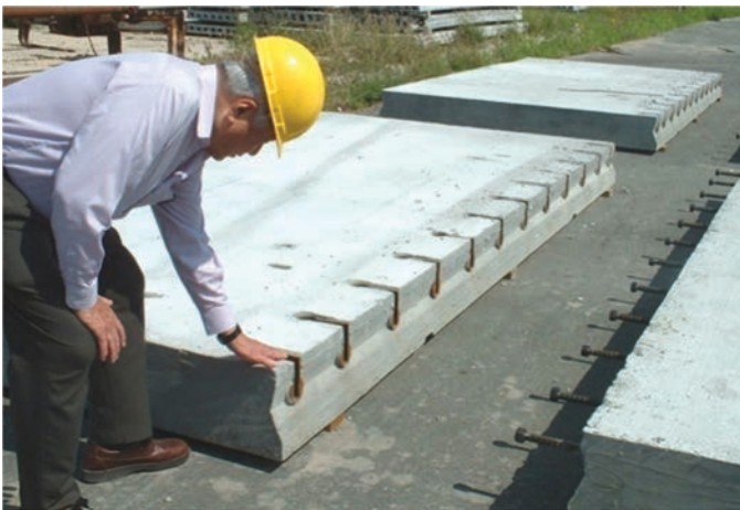
Figure 2.12. Kwik Slab joint interlocking system.
