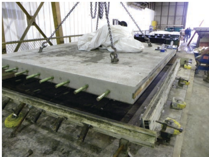
Figure 4.2. Typical four-point lifting of a precast panel.
