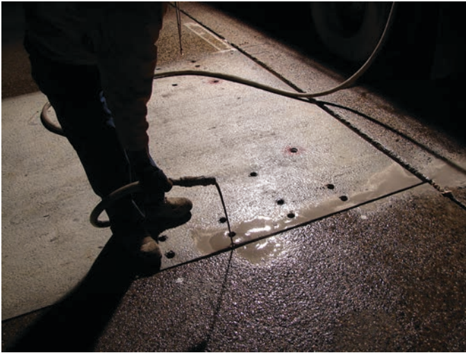
Figure 10.7. Dowel slot grouting.
