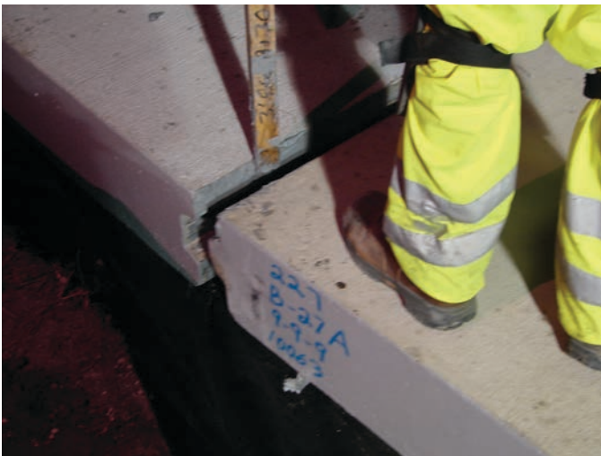
Figure 12.5. Intermediate keyway joint.
