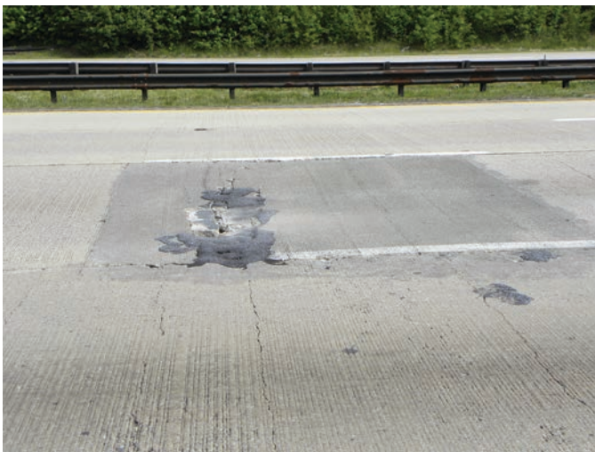
Figure 14.3. Failed FDRs in CRCP.
