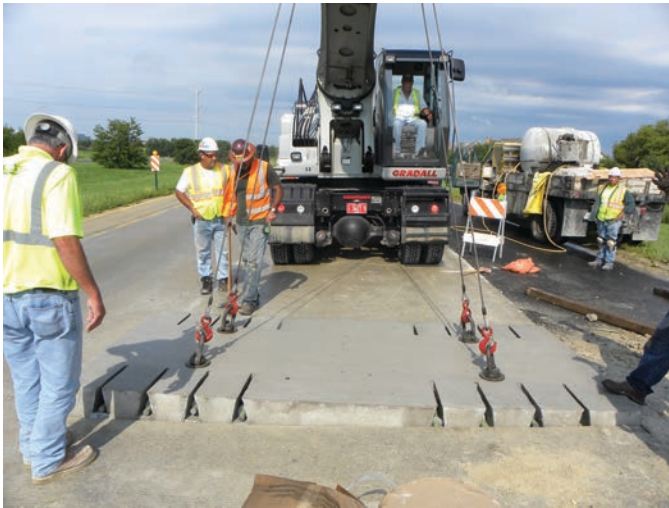
Figure 14.5. Narrow-mouth surface dowel slots.
