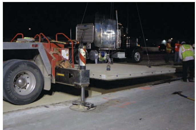
Figure 4.4. Outrigger positioning of lifting crane.
