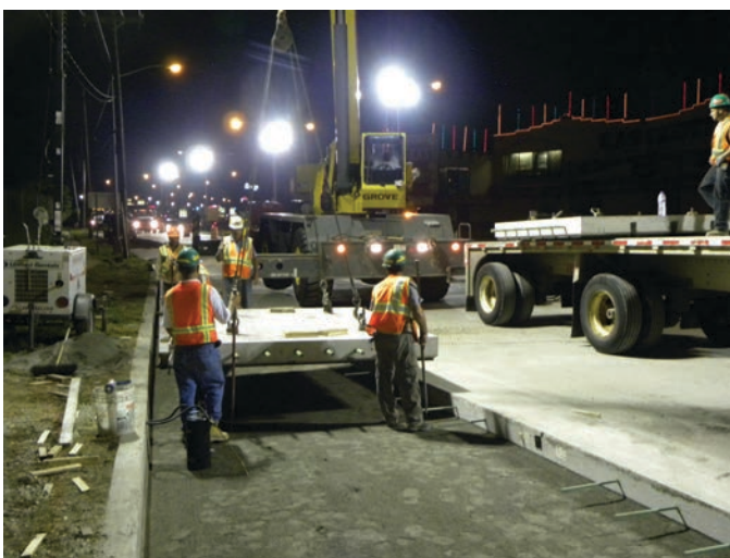
Figure 15.1. PCP installation at an intersection along Rockaway Boulevard in New York.
