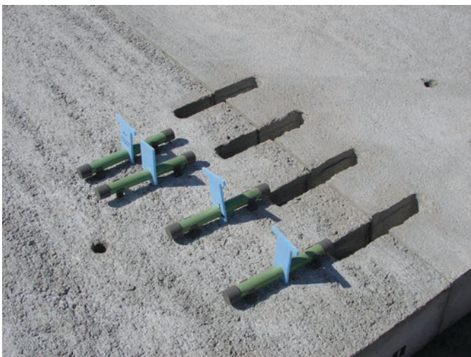
Figure 10.8. Slot patching for DBR.
