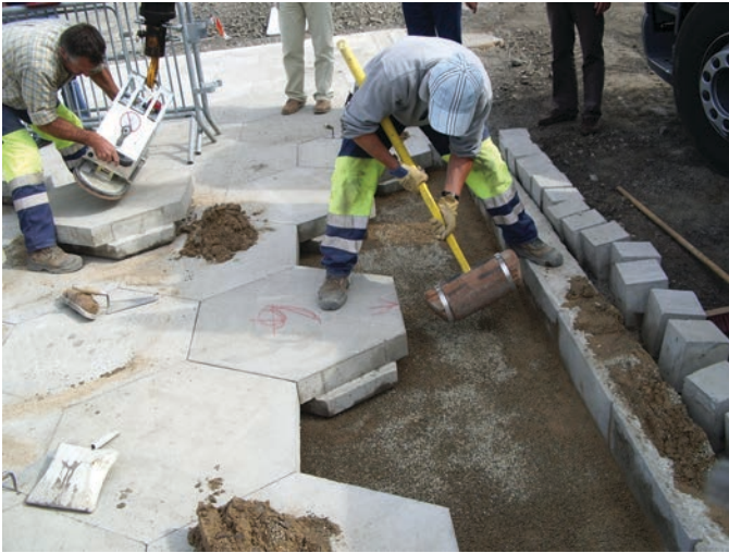
Figure 2.17. Installation of keyed hexagonal panels in France.
