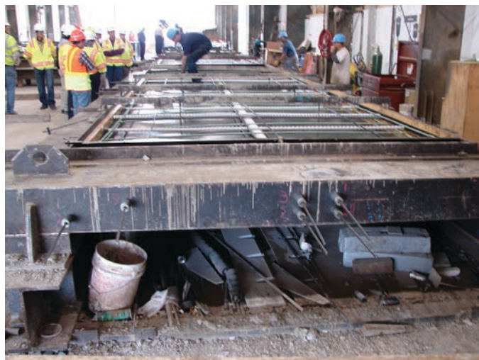
Figure 9.8. Pretensioning process.
