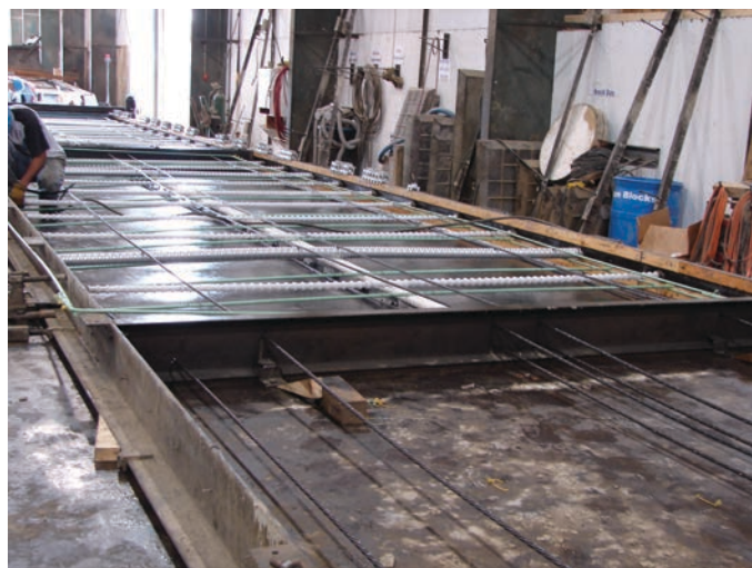
Figure 9.2. Formwork modified to allow for pretensioning strands.
