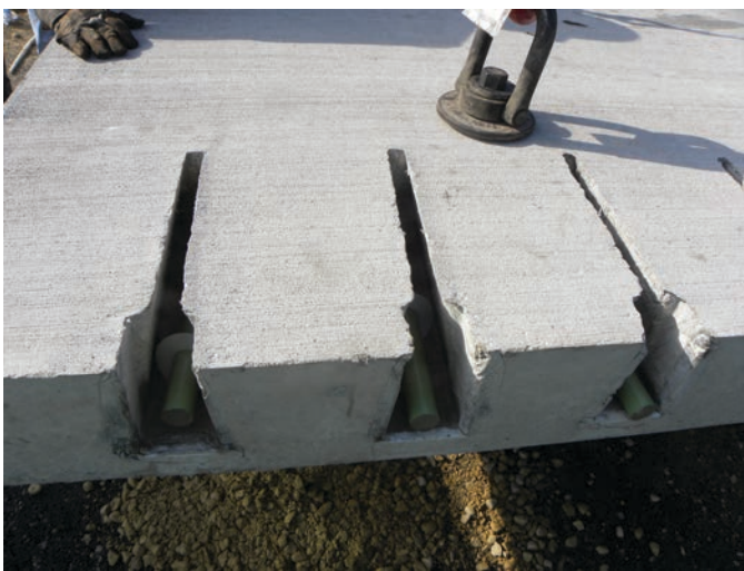
Figure 14.8. Three versions of the sliding dowel bar technique used in a 2011 Illinois Tollway demonstration project.
