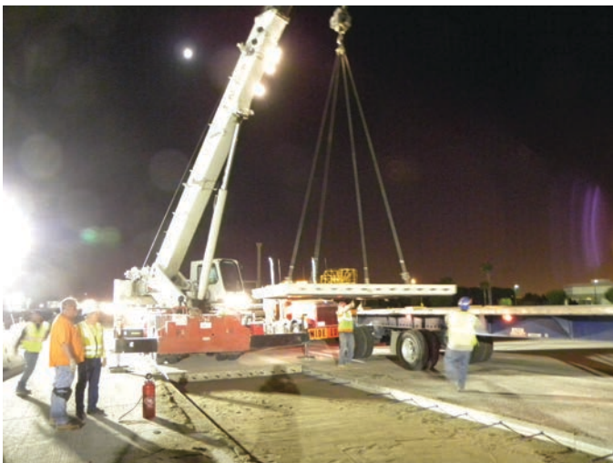
Figure 15.5. Typical panel-lifting equipment.
