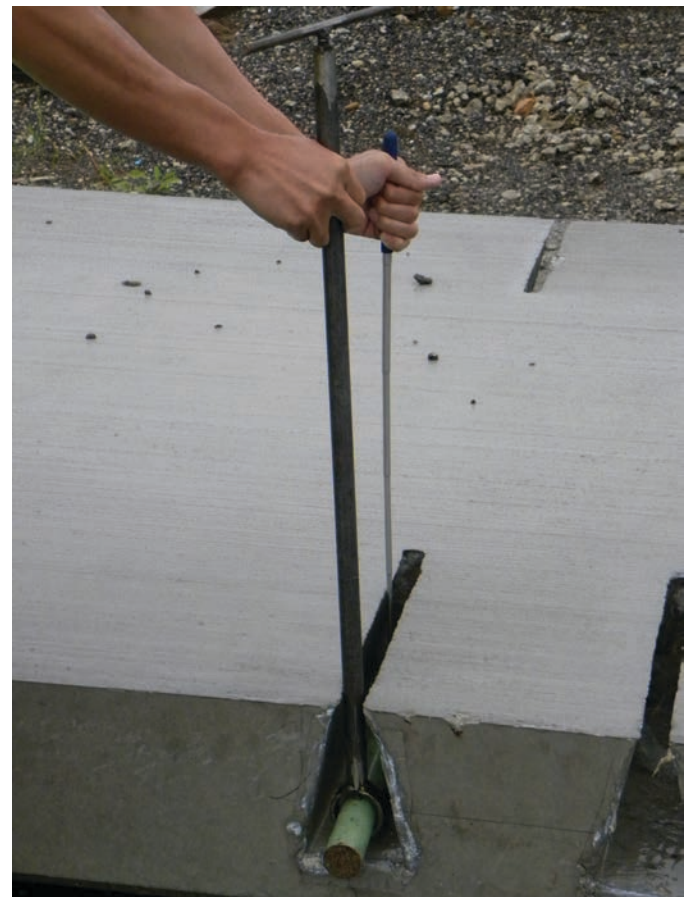
Figure 14.10. Tools to facilitate sliding the dowel bars in the slots and holding the bars in place.
