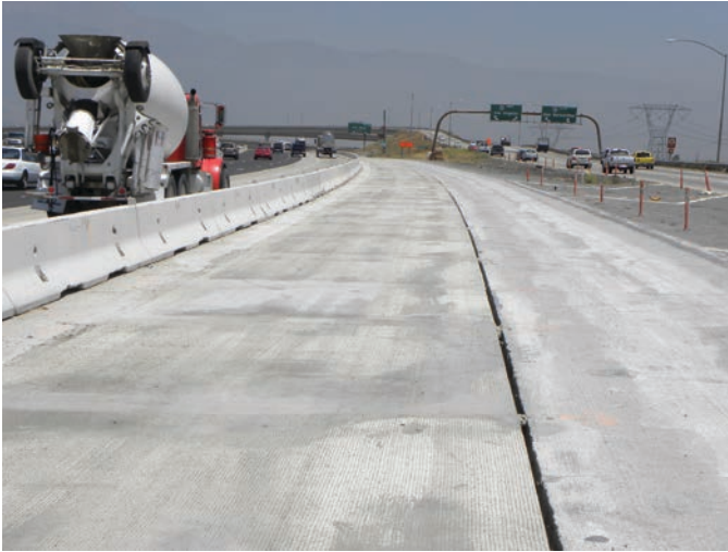
Figure 3.12. View of the I-15 JPrCP project in California.
