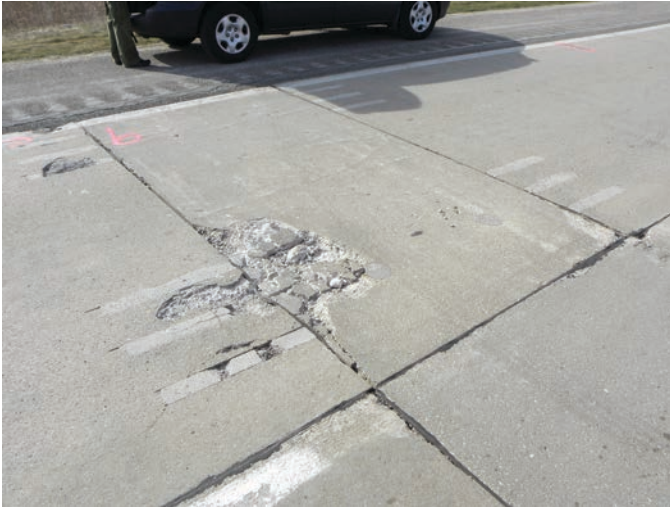
Figure 3.6. Views of a deteriorated panel at the I-675 project (planned for replacement) in Michigan.
