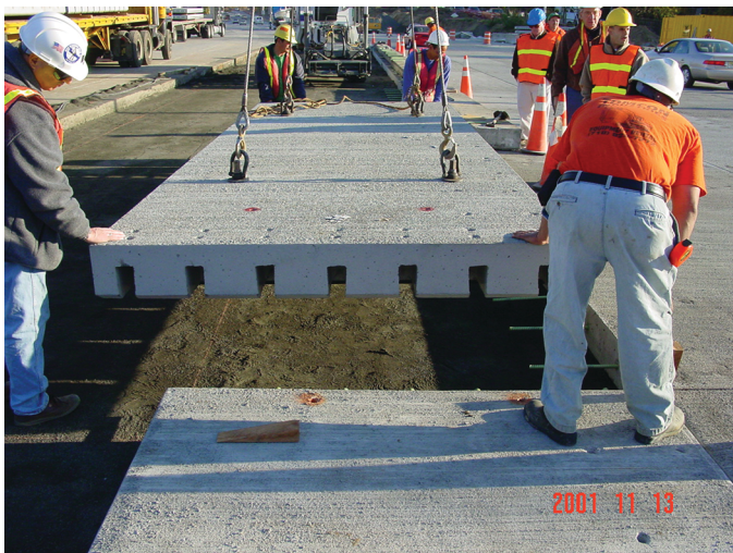
Figure 2.6. A scheme for providing load transfer in JPrCP using dowel slots and embedded dowel bars.
