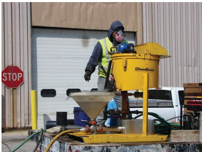
Figure 10.9. Undersealing grout pump and grouting operation.
