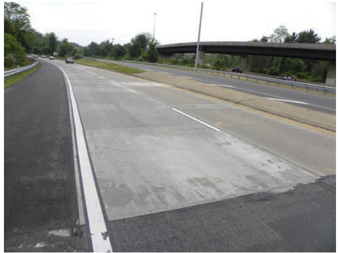
Figure 3.10. View of the I-66 JPrCP project in Virginia.
