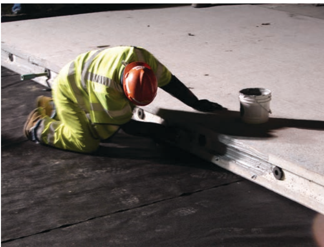
Figure 12.3. Applying epoxy along the transverse keyway joint face.
