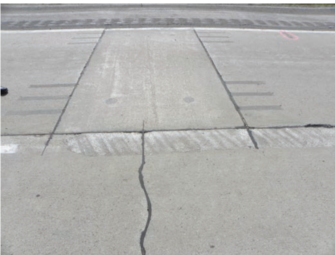
Figure 3.7. View of a well-performing panel at the I-675 project in Michigan.
