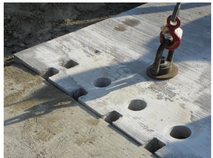
Figure 14.8. Three versions of the sliding dowel bar technique used in a 2011 Illinois Tollway demonstration project.
