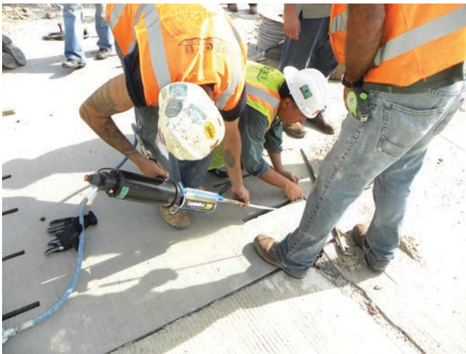
Figure 14.6. Narrow-mouth dowel slot use for repair applications.
