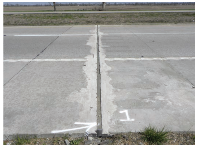
Figure 3.18. PPCP-reconstructed expansion joint on I-57 in Missouri.
