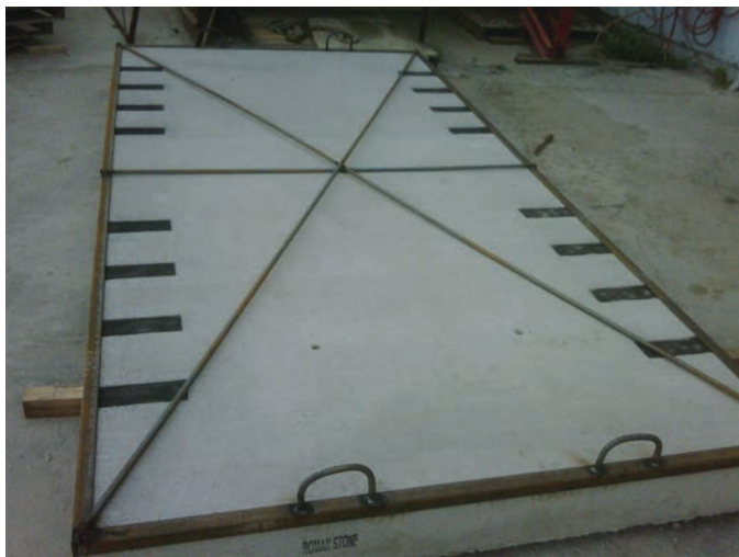
Figure 10.1. Template used for marking the repair area perimeter.
