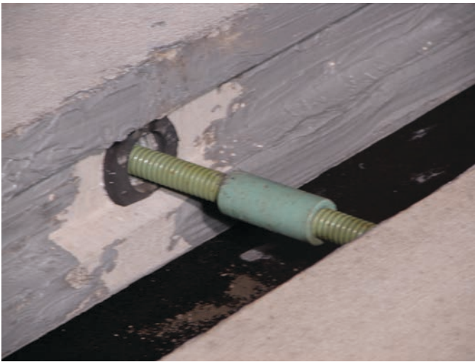
Figure 12.4. Gasket placed on tendon duct.
