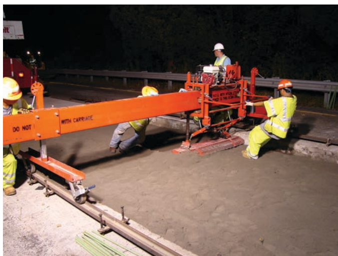
Figure 11.1. Manual base grading.
