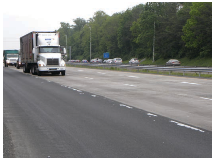
Figure 3.22. View of the I-66 PPCP project in Virginia.
