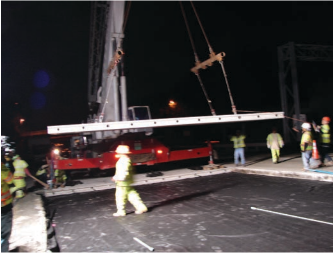
Figure 12.2. Panel placement.
