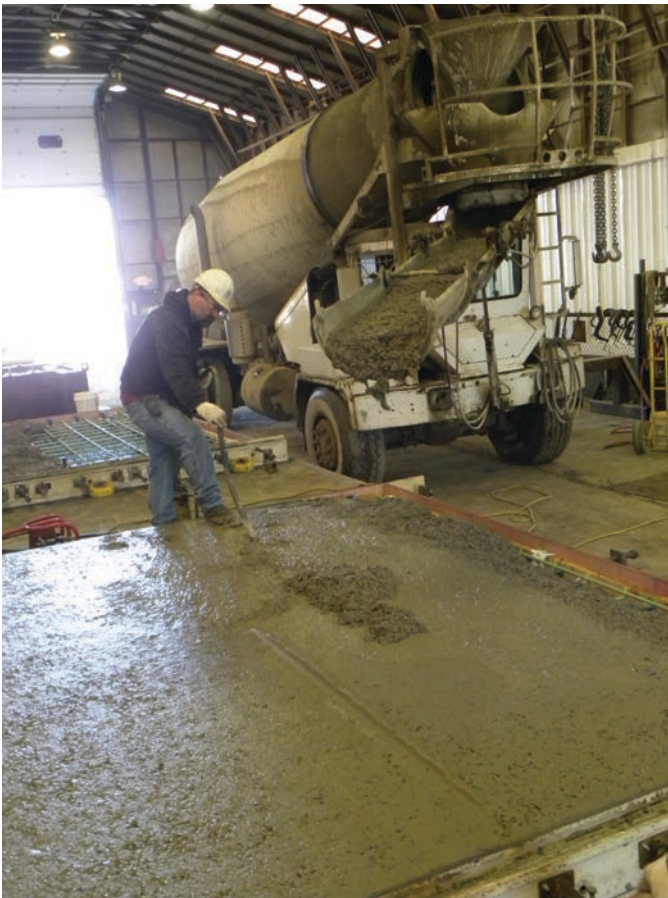
Figure 9.6. Concrete delivery options (transit mixer and bucket).
