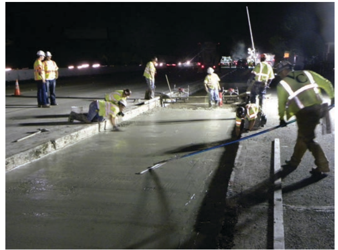
Figure 11.2. Material being directly deposited in PPCP work areas: (left) CTPB placement during Delaware project and (right) LCB placement during California I-680 project.
