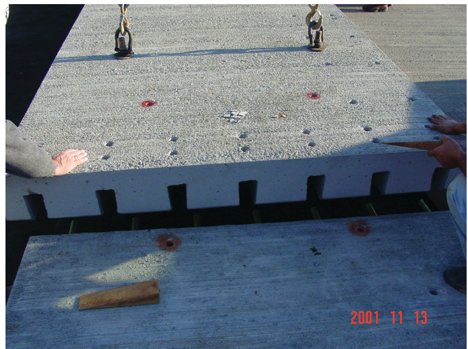
Figure 2.6. A scheme for providing load transfer in JPrCP using dowel slots and embedded dowel bars.
