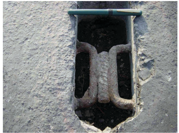
Figure 2.15. Soviet-era precast panels (left) and lifting loops with reinforcing bar (right).
