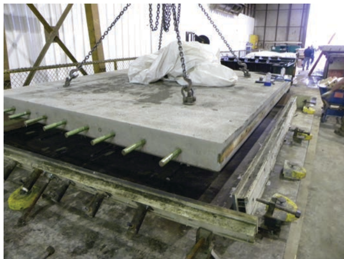
Figure 9.9. Stripped panel being moved to another location and panel with project-specific markings.
