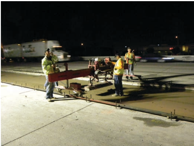
Figure 15.3. Lane closure scenario for a continuous PCP application.
