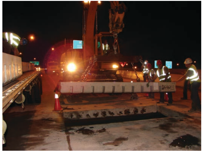
Figure 15.2. Crane placement of panel on four-lane divided highway project.
