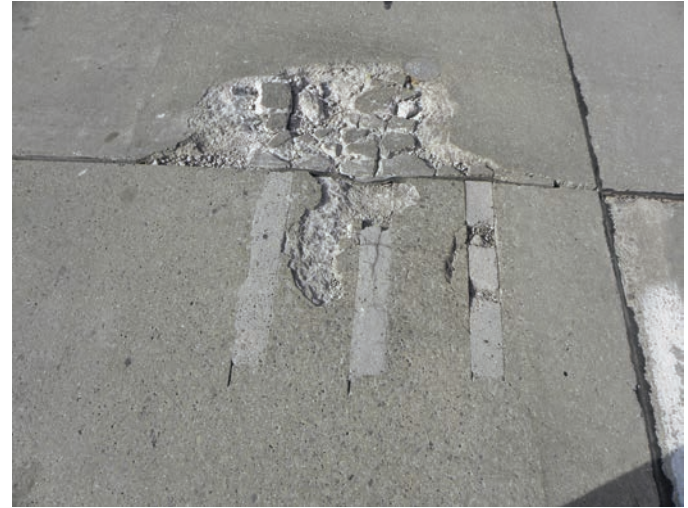
Figure 3.6. Views of a deteriorated panel at the I-675 project (planned for replacement) in Michigan.
