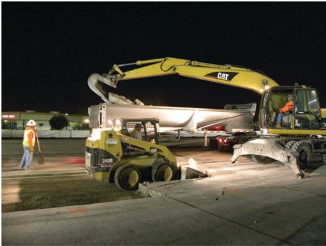
Figure 15.2. Crane placement of panel on four-lane divided highway project.
