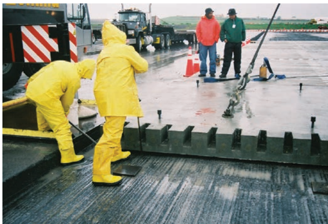
Figure 2.7. An alternate scheme for providing load transfer in JPrCP.
