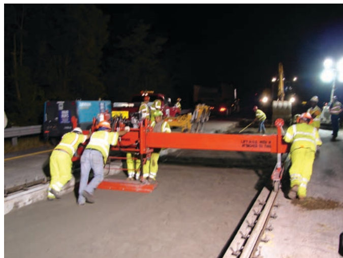
Figure 6.1. Auger-based granular base grading system.
