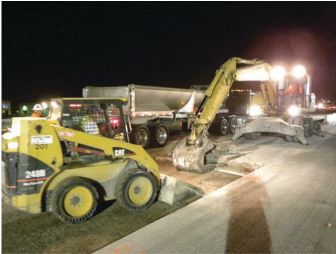
Figure 15.4. Different types of pavement removal equipment.
