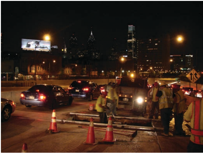
Figure 15.2. Crane placement of panel on four-lane divided highway project.
