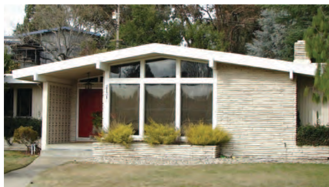
Figure 97. Concrete screen at the front entrance of a c.1964 Ranch house in Sacramento, California (photograph courtesy of Andrew Hope, Caltrans).
