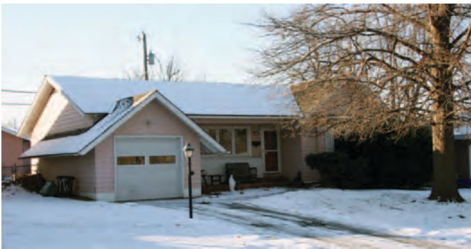
Figure 32. Storybook style house in Omaha, Nebraska (locally referred to as a Chalet Ranch), constructed c.1950, that has sweeping gables and non-compatible replacement vinyl siding and windows. As a result, it does not meet the survey criteria due to the lack of historic integrity (Mead & Hunt photograph).
