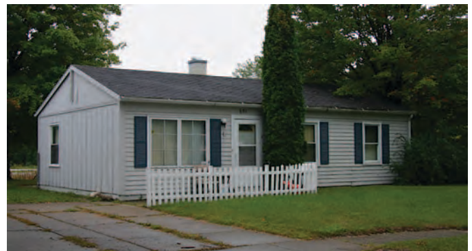
Figure 167. National Homes prefabricated house in the Snyder Subdivision in Mason, Michigan, erected c.1956, with replacement siding and windows (Mead & Hunt photograph).
