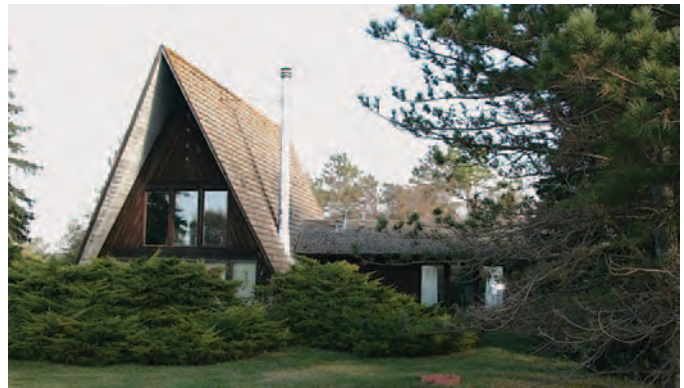
Figure 158. A-frame house in Overton, Nebraska, constructed c.1970, with overhanging eaves and a one-story addition on the side (Mead & Hunt photograph).
