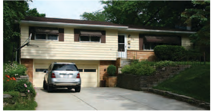
Figure 131. Raised Ranch in Madison, Wisconsin, constructed c.1960, with a partially exposed basement, integrated garage, picture window, overhanging eaves, wide chimney, and accent brick veneer (Mead & Hunt photograph).
