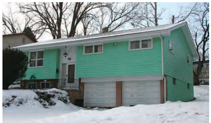
Figure 140. Split-foyer house in Omaha, Nebraska, constructed c.1965, with a central exaggerated-height entrance, two levels of living space, accent brick veneer, and an integrated basement-level garage (Mead & Hunt photograph).
