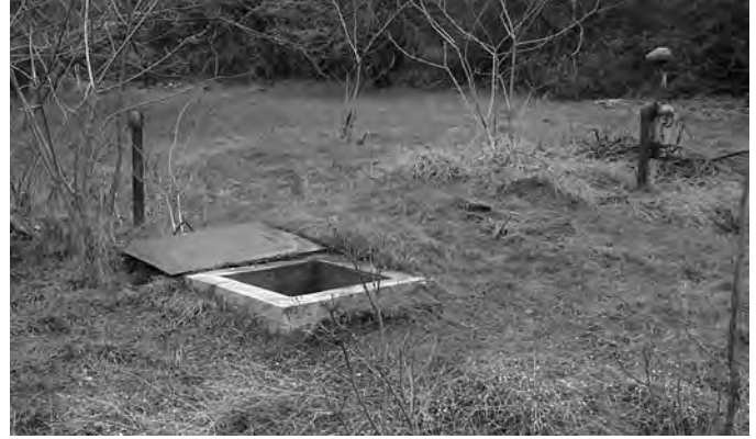
Figure 176. Bomb shelter in Sonora, California, constructed c. 1960, from left to right are the exhaust air vent, hatch, and fresh air intake (photograph courtesy of Andrew Hope, Caltrans).
