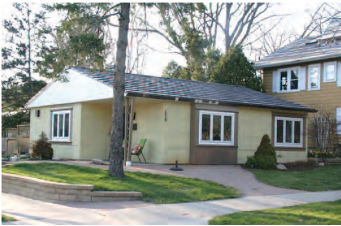
Figure 163. Lustron house in Madison, Wisconsin, erected c.1950, retains the porcelain enamel maize yellow siding, steel roof, and inset entry and support post; the windows have been replaced (Mead & Hunt photograph).
