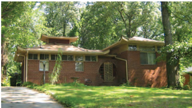
Figure 152. Asiatic style applied to the Split-level form in the Collier Heights Historic District in Atlanta, Georgia, with upturned eaves and an Asian-inspired entrance (photograph courtesy of Sandy Lawrence, Georgia Department of Transportation).
