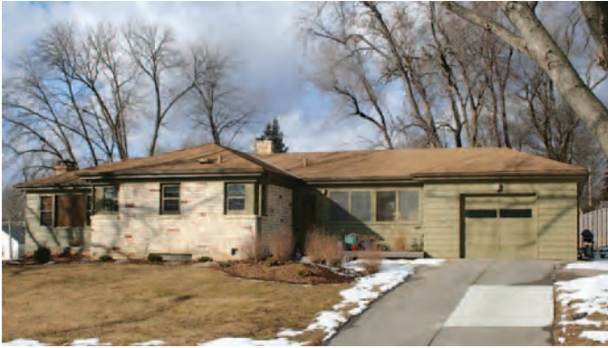
Figure 125. Ranch house in Omaha, Nebraska, constructed c.1955, with horizontal massing, hip roof, clapboard and stone veneer, picture and double-hung windows, and attached breezeway and garage (Mead & Hunt photograph).
