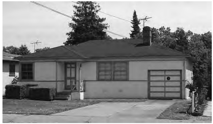
Figure 121. Transitional Ranch in San Lorenzo, California, with compact massing, integrated garage, and recessed entrance. The house was constructed by merchant builder Dave Bohannon c.1950 (photograph courtesy of Andrew Hope, Caltrans).
