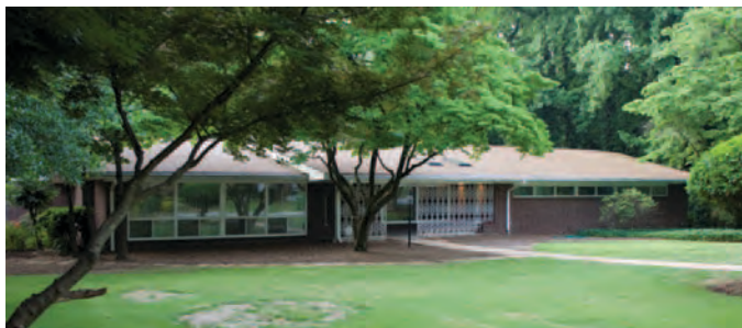
Figure 48. Hermann J. Russell Ranch house, constructed in 1963 and located in the National Register-listed Collier Heights Historic District in Atlanta, Georgia (photograph courtesy of Georgia Department of Natural Resources, Historic Preservation Division).
