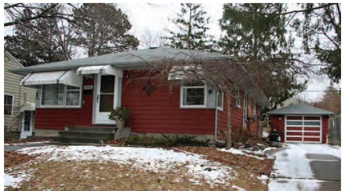
Figure 122. Transitional Ranch in St. Louis Park, Minnesota, constructed c.1950, with compact massing, corner windows, low-pitched roof with a wide eave overhang, and attached garage at the rear (Mead & Hunt photograph).
