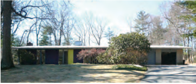
Figure 92. ALCOA Care-free House in Lincoln, Massachusetts, with a white anodized standing seam roof, purple anodized corrugated wall panels, and anodized yellow door cladding (photograph courtesy of John A. Burns, FAIA).
