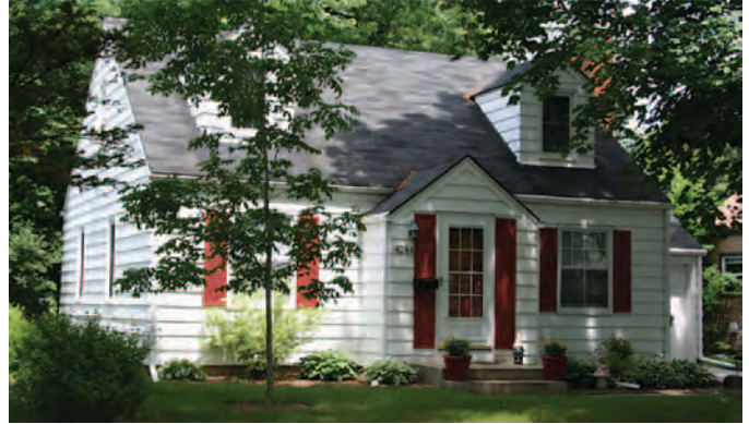
Figure 11. Cape Cod house in Madison, Wisconsin, constructed c.1945, retains its original massing, siding, windows, and entrance, and thus meets the survey criteria (Mead & Hunt photograph).
