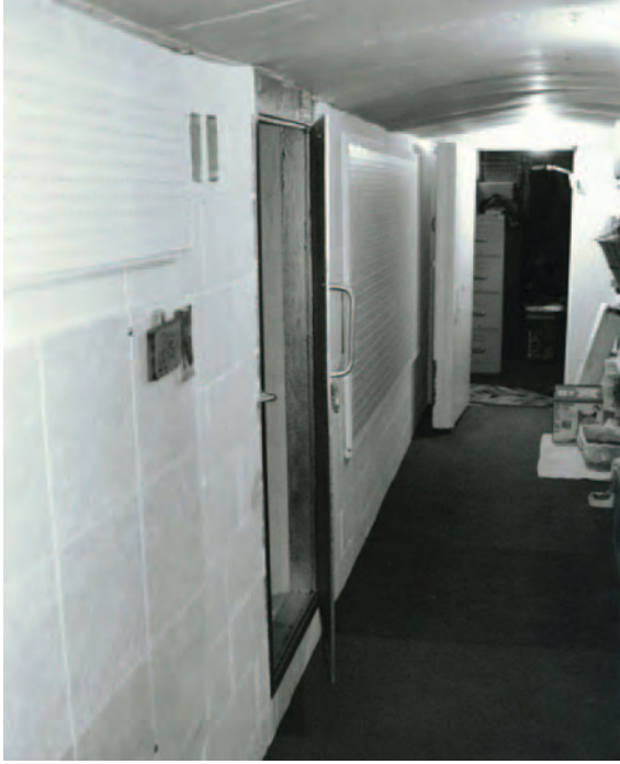
Figure 175. Concrete tunnel between the Gainsforth House and garage in Ogallala, Nebraska, that also led to the family bunker (photograph courtesy of the Nebraska State Historical Society).
