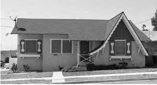
Figure 146. This house in San Diego, California, constructed c.1957, displays the Ranch form and Storybook features, including scalloped barge boards, diamond-pane windows, decorative shutters and planter boxes, and a sweeping gable (photograph courtesy of Andrew Hope, Caltrans).
