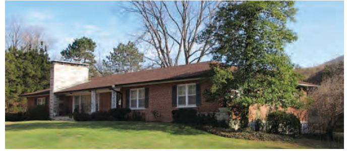
Figure 129. Ranch house in Richmond Heights, Missouri, with horizontal massing, hip roof, integrated stone planters, prominent stone chimney, and wrought iron supports at the entrance (photograph courtesy of Toni Prawl, Missouri Department of Transportation).
