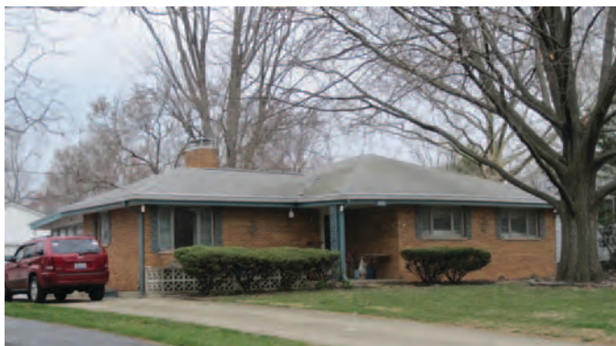
Figure 103. Ranch house in Upper Arlington, Ohio, constructed c.1955, with a hip roof, brick veneer, recessed entrance with decorative wrought iron details, and decorative shutters (Mead & Hunt photograph).
