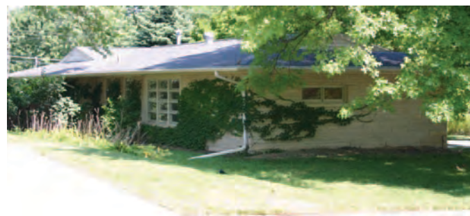
Figure 101. Grouping of 12 Flexivent windows on the rear elevation of a c.1953 Ranch home in Lincoln, Nebraska (Mead & Hunt photograph).
