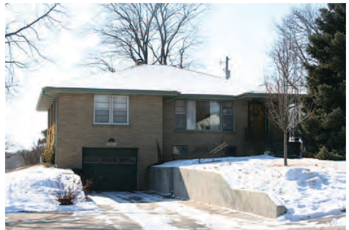
Figure 132. Raised Ranch in Omaha, Nebraska, constructed c.1955, with a partially exposed basement, integrated garage, picture and double-hung windows, overhanging eaves, and wrought iron details at the entrance (Mead & Hunt photograph).
