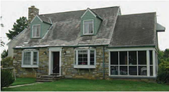
Figure 115. Cape Cod house in Arlington County, Virginia, constructed c.1950, with one-and-one-half-story massing, side gable roof with twin dormers, stone veneer, and sun porch (Mead & Hunt photograph).
