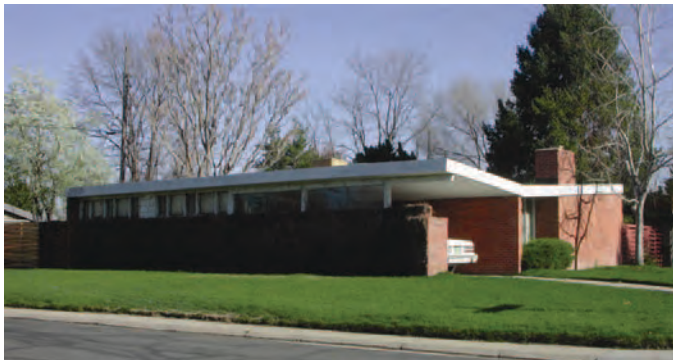
Figure 62. Contemporary style house with an integrated carport in the Arapahoe Acres Historic District in Englewood, Colorado (photograph courtesy of Diane Wray Tomasso).
