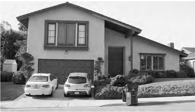
Figure 136. Split-level house in San Diego, California, constructed c.1968, with clearly zoned wings on different levels opening off the centrally located entry, casement windows, and an integrated garage (photograph courtesy of Andrew Hope, Caltrans).
