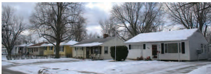
Figure 8. Modified Gunnison houses in the Maenner South Addition in Omaha, Nebraska. This streetscape documents the similar form and massing and setbacks within the addition (Mead & Hunt photograph).
