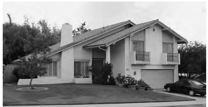
Figure 150. Spanish Colonial Revival style applied to the Split-level form in La Mesa, California, constructed c.1970, with stucco exterior and tile roof (photograph courtesy of Andrew Hope, Caltrans).
