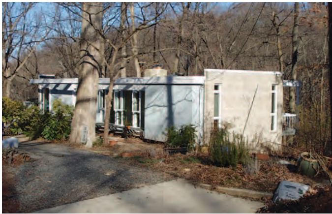
Figure 15. A Contemporary-style house located at 3710 30th Street North in Bellevue Forest, built in 1963 (Louis Berger photograph).
