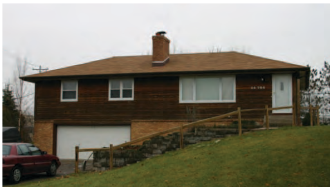
Figure 22. Raised Ranch house in Hennepin County, Minnesota, with non-compatible replacement wood siding and only two architectural elements: accent brick veneer and the prominent chimney. As a result, it does not meet the survey criteria (Mead & Hunt photograph).
