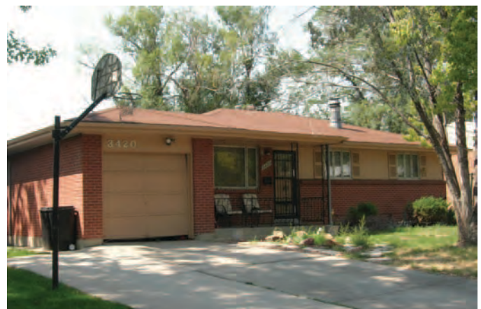
Figure 102. Ranch house in Westminster, Colorado, with a hip roof, partial brick veneer, recessed entrance with decorative wrought iron details, and decorative shutters (photograph courtesy of Dianna Litvak, Colorado Department of Transportation).
