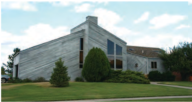
Figure 156. Shed house in Lexington, Nebraska, constructed c.1975, with geometric massing, prominent shed roof lines, natural wood siding, and minimal exterior decoration (Mead & Hunt photograph).
