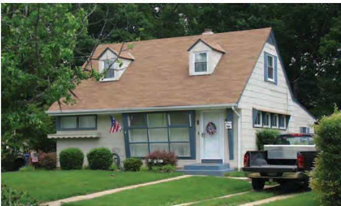
Figure 117. Cape Cod house in Fairfax County, Virginia, with one-and-one-half-story massing, side gable roof with twin dormers, and canted front picture window (photograph courtesy of Anne Bruder, Maryland State Highway Administration).
