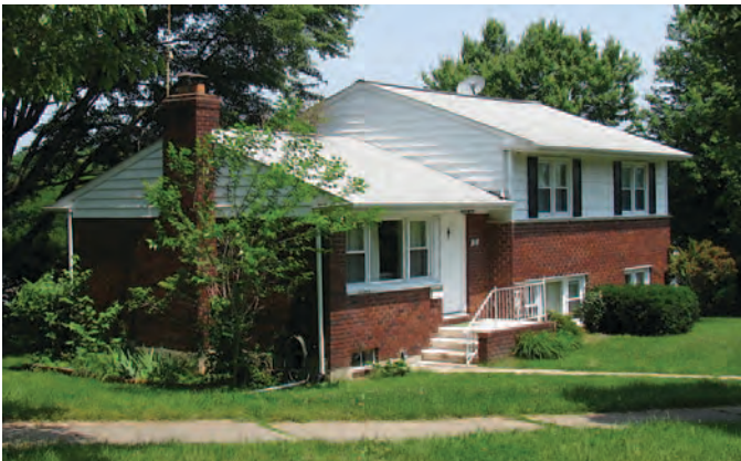
Figure 138. Split-level house in Baltimore County, Maryland, with an elevated entry, brick veneer, and picture window (photograph courtesy of Anne Bruder, Maryland State Highway Administration).
