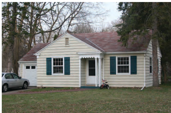
Figure 112. Minimal Traditional house in Madison, Wisconsin, constructed c.1945, with wood siding, compact one-story plan, minimal eave overhang, inset entrance, attached one-car garage, and modest Colonial Revival details, including gable end returns and cornice boards (Mead & Hunt photograph).
