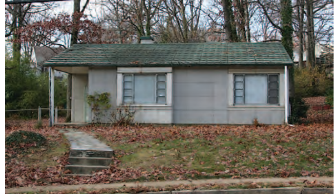
Figure 162. Lustron house in Arlington County, Virginia, erected in 1949, retains the porcelain enamel dove gray siding, steel roof, inset entry and support post, and steel windows (Mead & Hunt photograph).
