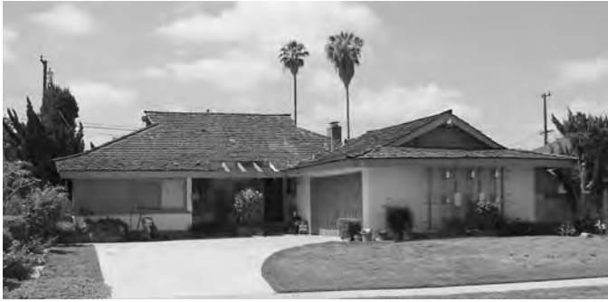
Figure 151. Asiatic style applied to the Ranch form in Whittier, California, constructed c.1960, with exaggerated eaves and a decorative screen (photograph courtesy of Andrew Hope, Caltrans).
