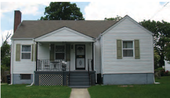
Figure 10. Minimal Traditional house in Prince George's County, Maryland, constructed c.1945, with non-compatible vinyl siding, replacement windows, and a modified stoop. As a result, it does not meet the survey criteria (photograph courtesy of Anne Bruder, Maryland State Highway Administration).
