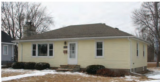
Figure 14. Transitional Ranch house in St. Louis Park, Minnesota, constructed in 1953, does not meet the survey criteria due to the replacement vinyl siding and windows (Mead & Hunt photograph).
