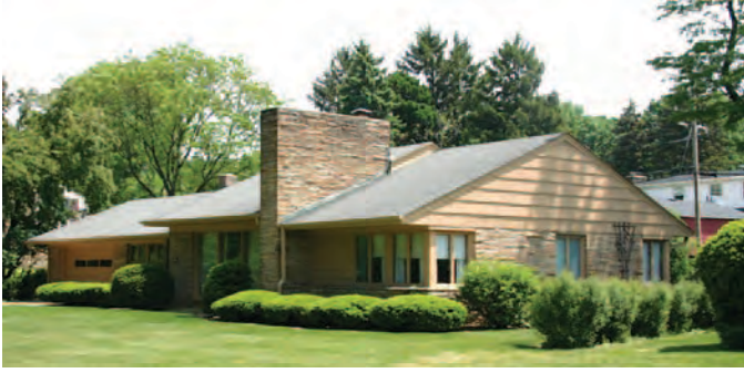
Figure 16. Ranch house in Milwaukee, Wisconsin, constructed c.1960, retains multiple architectural elements, including accent wood shingle siding, prominent wide chimney, and corner windows, and thus meets the survey criteria (Mead & Hunt photograph).
