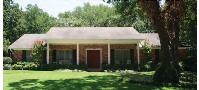
Figure 142. Ranch house in Arlington, Texas, constructed in 1966, displays elements of the Colonial Revival style, including symmetrical massing and wide porch with turned columns (Mead & Hunt photograph).
