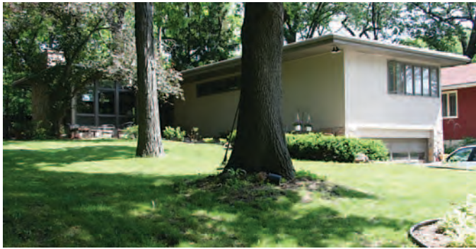
Figure 169. Prefabricated U-Form-It House in Madison, Wisconsin, erected in 1955 (Mead & Hunt photograph).
