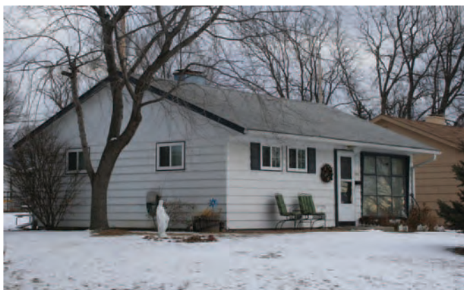
Figure 55. Prefabricated Gunnison Homes residence in Omaha, Nebraska, erected c.1955, that individually does not represent innovations in postwar residential prefabrication since the construction materials were already widely accepted (Mead & Hunt photograph).
