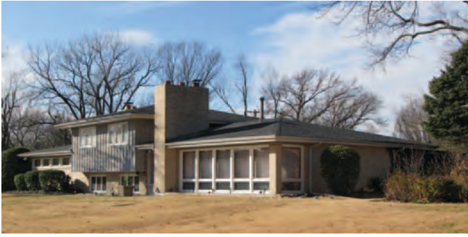
Figure 24. Split-level residence in Richmond Heights, Missouri, retains its original form, and displays multiple architectural elements, including accent board and batten siding, prominent chimney, and bands of windows. As a result, it meets the survey criteria (photograph courtesy of Toni Prawl, Missouri Department of Transportation).
