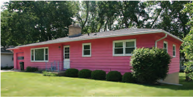
Figure 17. Ranch house in Madison, Wisconsin, constructed in 1958, retains its original massing, siding, and window configuration but does not display three architectural elements and does not meet the survey criteria (Mead & Hunt photograph).
