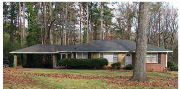
Figure 130. Ranch house in De Kalb County, Georgia, constructed c.1955, with horizontal massing, hip roof, accent stone veneer, breezeway, and concrete screening at the carport (photograph courtesy of Georgia Department of Natural Resources, Historic Preservation Division).
