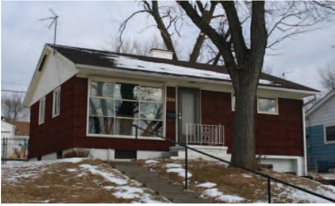
Figure 37. Prefabricated U.S. Steel home in Omaha, Nebraska, constructed in 1955, retains its original footprint, windows, and cladding materials, and thus meets the survey criteria (Mead & Hunt photograph).
