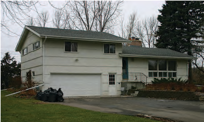
Figure 137. Split-level house in Hennepin County, Minnesota, constructed c.1965, with an elevated entry, integrated garage, slab chimney, and multi-light picture window (Mead & Hunt photograph).
