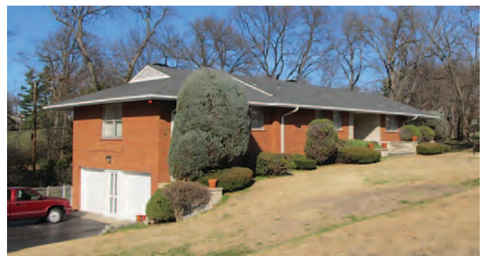
Figure 133. Raised Ranch house in Richmond Heights, Missouri, with the exposed basement at the side elevation, accent stone veneer, and planters (photograph courtesy of Toni Prawl, Missouri Department of Transportation).
