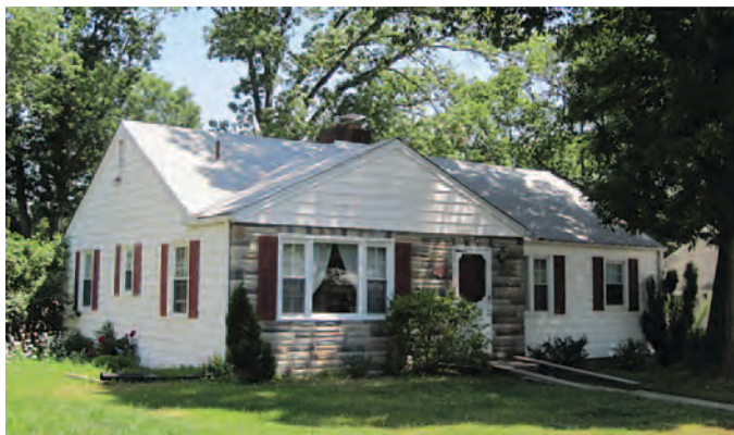
Figure 9. This house in Virginia Heights, built in 1950, is clad with Formstone, a non-traditional material introduced on Arlington houses in the 1950s (Mead & Hunt photograph).
