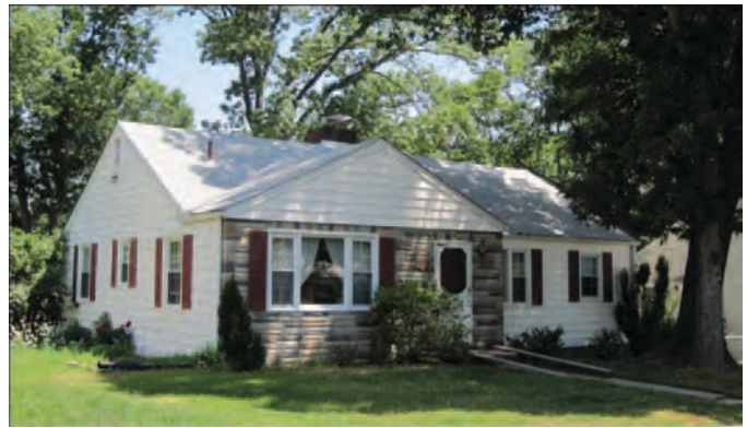
Figure 64. Minimal Traditional house, constructed in 1950, with wide-lap replacement vinyl siding that visually imitates original materials in the National Register-listed Virginia Heights Historic District in Arlington County, Virginia (Mead & Hunt photograph).
