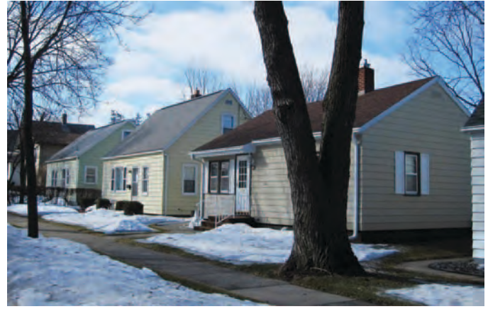
Figure 94. Three c.1945 Minimal Traditional residences in St. Cloud, Minnesota, with aluminum siding (Mead & Hunt photograph).
