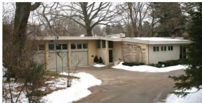
Figure 69. Contemporary residence in Omaha, Nebraska, constructed in 1954, with a modern three-car garage that replaced the historic carport; this alteration compromises the integrity, and the property is considered not individually eligible (Mead & Hunt photograph).
