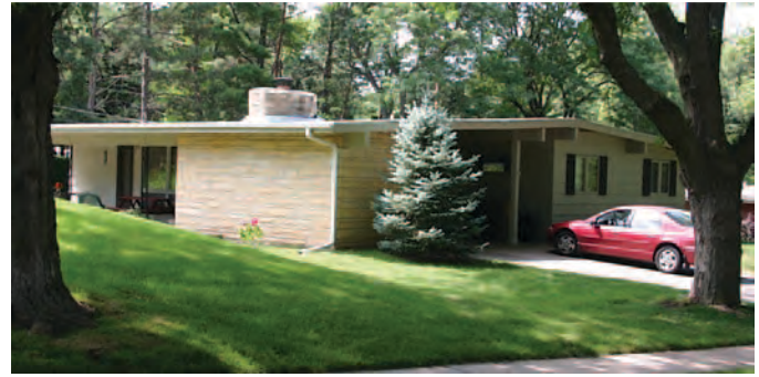
Figure 172. Patio located at rear elevation of c.1956 Ranch house in Lincoln, Nebraska (Mead & Hunt photograph).
