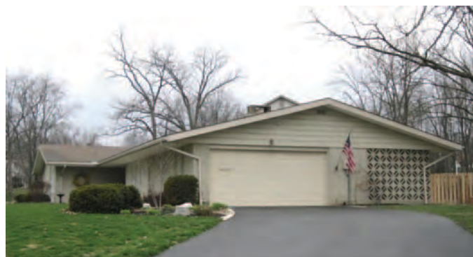
Figure 96. Concrete screen providing increased privacy at the rear patio of this c.1966, Worthington Hills, Ohio, Ranch house (Mead & Hunt photograph).
