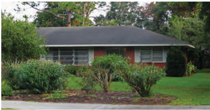
Figure 105. Awning-style windows grouped to form a picture window on a Jekyll Island, Georgia, Ranch house (photograph courtesy of Georgia Department of Natural Resources, Historic Preservation Division).
