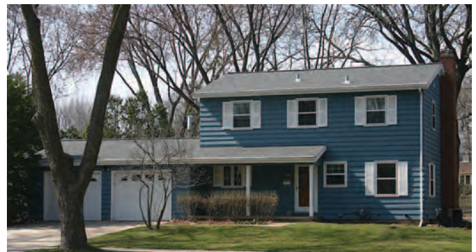
Figure 120. Two-story Massed house in Madison, Wisconsin, constructed in 1959, featuring a rectangular plan, two-story massing, and side gable roof (Mead & Hunt photograph).
