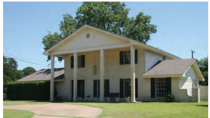
Figure 27. Colonial Revival in Arlington, Texas, constructed in 1967, retains its original materials and massing and displays multiple architectural elements, including a decorative door surround, projecting front gable, and compass vent. As a result, it meets the survey criteria (Mead & Hunt photograph).
