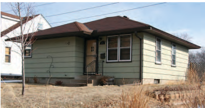
Figure 4. Intact c.1950 house in the postwar St. Louis Park, Minnesota, neighborhood. This residence represents the Transitional Ranch form. The house retains the original footprint, wide-lap wood siding, and double-hung windows, which are partially obscured by modern storm windows (Mead & Hunt photograph).
