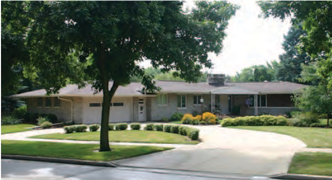
Figure 126. Ranch house in Sparta, Wisconsin, constructed c.1960, with horizontal massing, hip roof, stone veneer, casement windows, wrought iron supports at the entrance, prominent chimney, and attached garage. It is oriented diagonally on a large urban lot (Mead & Hunt photograph).
