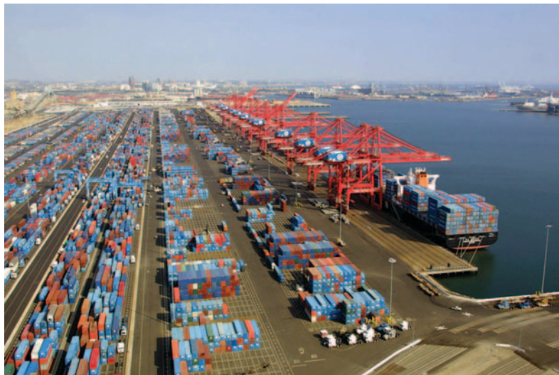
Figure 2-2. Grounded Operations at Hanjin Terminal, Port of Long Beach
