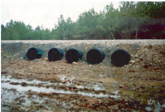
Figure 5-1. Example of multibarrel culvert installation.
