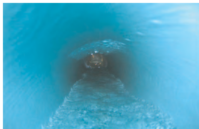
Figure 5-4. Example of surface waves inside the culvert.
