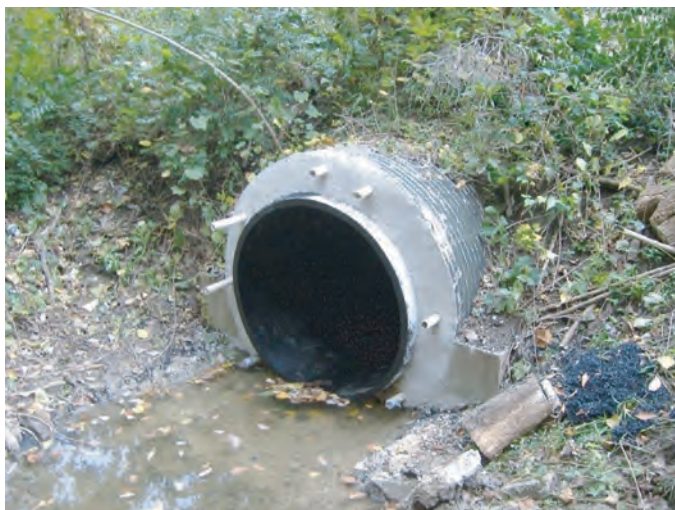
Figure 3-1. Example of a slip-lined culvert.
