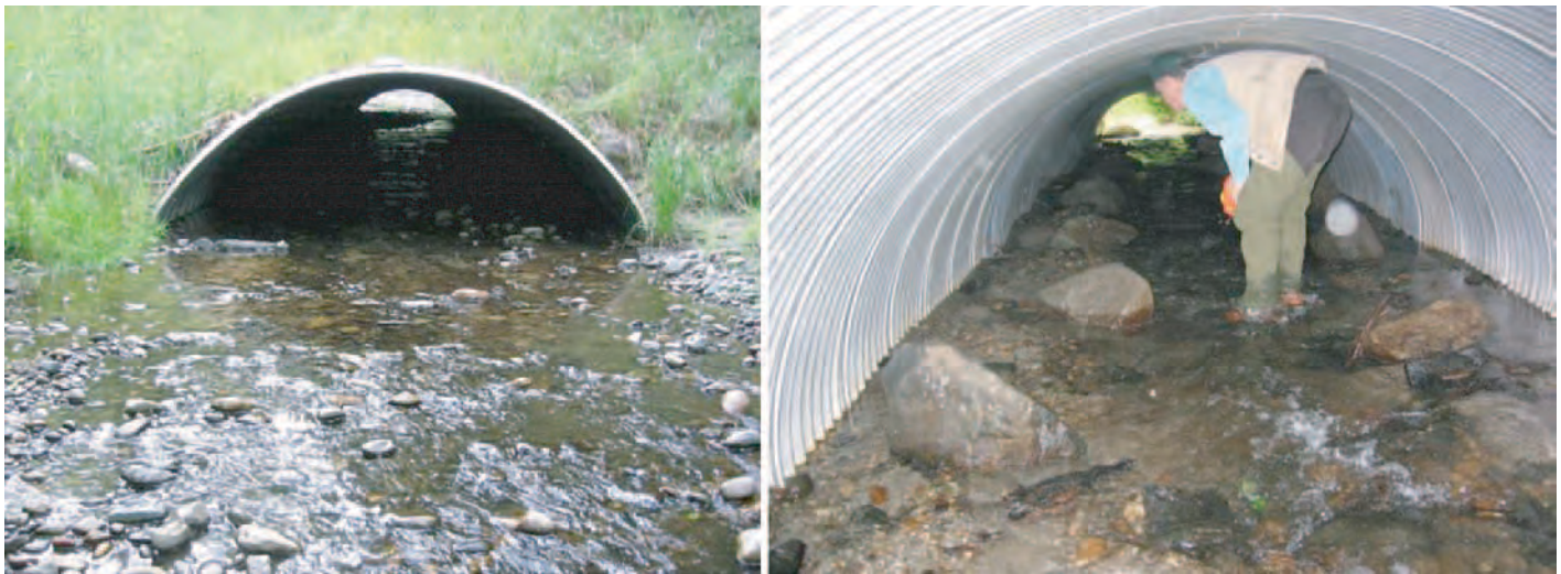
Figure 2-1. Examples of buried-invert culverts for fish passage.
