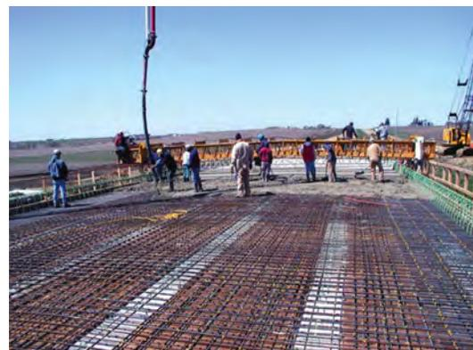
MMFX steel was used in the construction of a bridge deck in Gundy County, Iowa. The developer of the corrosion-resistant and high-strength material began experimenting with dual-phase ferritic martensitic reinforcing steel under an NCHRP IDEA project.
