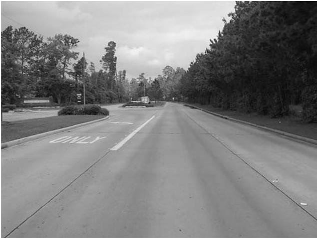
FIGURE 20 Median opening for left-turn lane on a four-lane divided suburban arterial at an unsignalized three-leg intersection (Credit: Dan Walker, Texas Transportation Institute).
