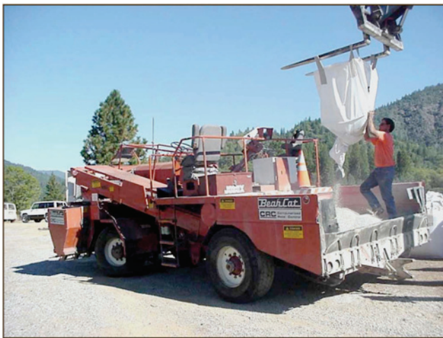
FIGURE 20 Chip spreader application of aggregates.
