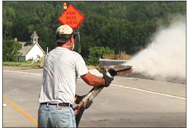
FIGURE 9 Equipment used to blow aggregates onto overlay surface.
