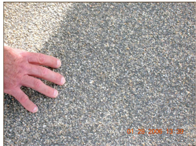
FIGURE 22 Finished overlay surface.
