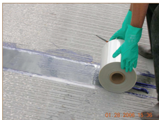
FIGURE 15 Fiber fabric applied previous to overlay over bridge joint.
