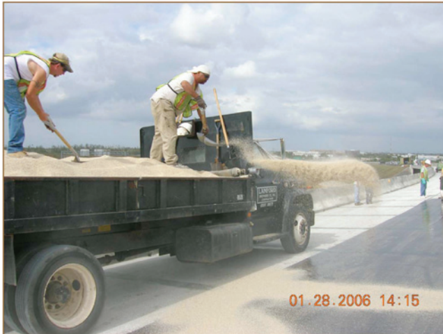
FIGURE 19 Hand application of aggregates over resin.
