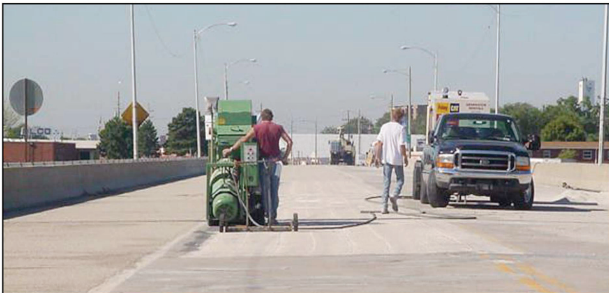
FIGURE 1 Shot-blast preparation of the surface.
