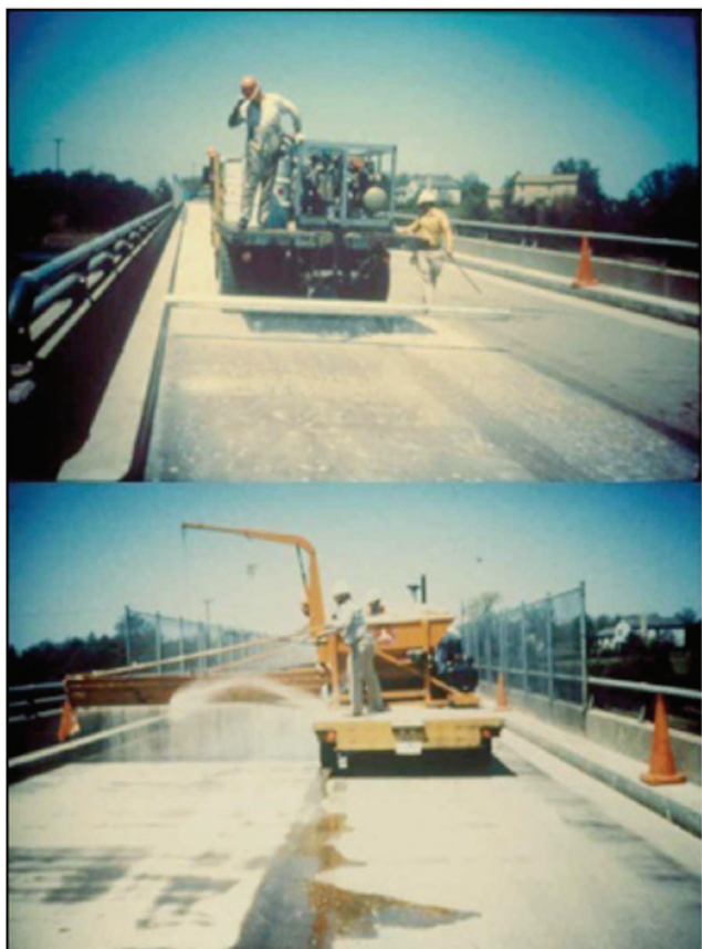
FIGURE 3 Workers spraying resin followed by application of aggregates in multiple-layer TPO.
