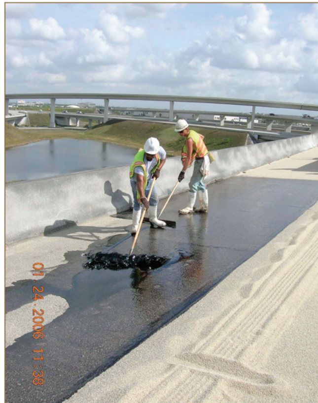
FIGURE 18 Brooming epoxy over surface.
