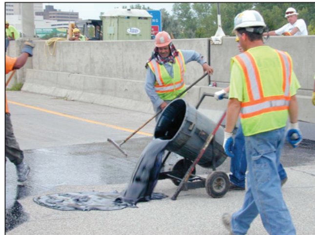
FIGURE 17 Applying epoxy to deck for multiple-layer overlay.
