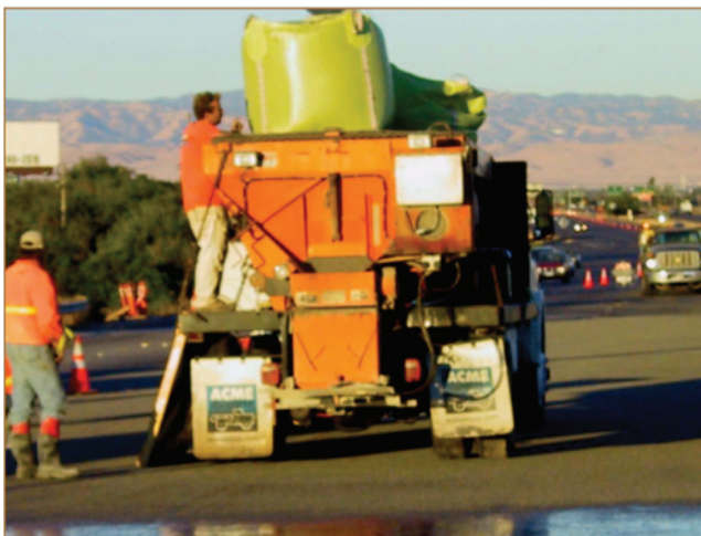
FIGURE 21 Salting truck for applying aggregates over epoxy.
