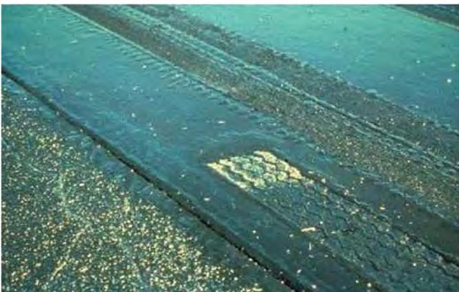
**Figure 19. Excessive tack coat spray application.**
