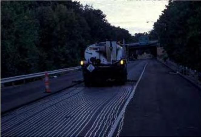
**Figure 16. Non uniform tack coat spray application—blocked and oversize nozzles.**
