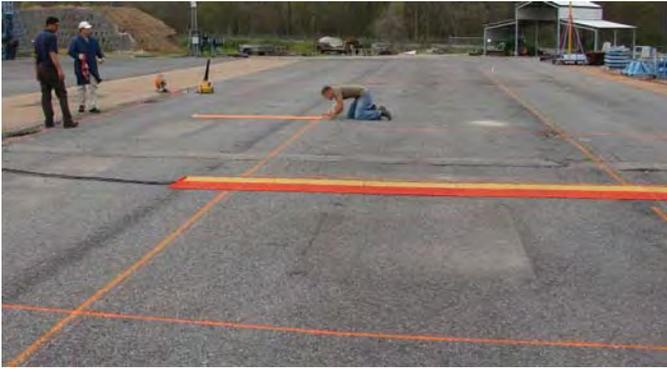
**Figure 12. Preparation of test lanes for tack coat application.**
