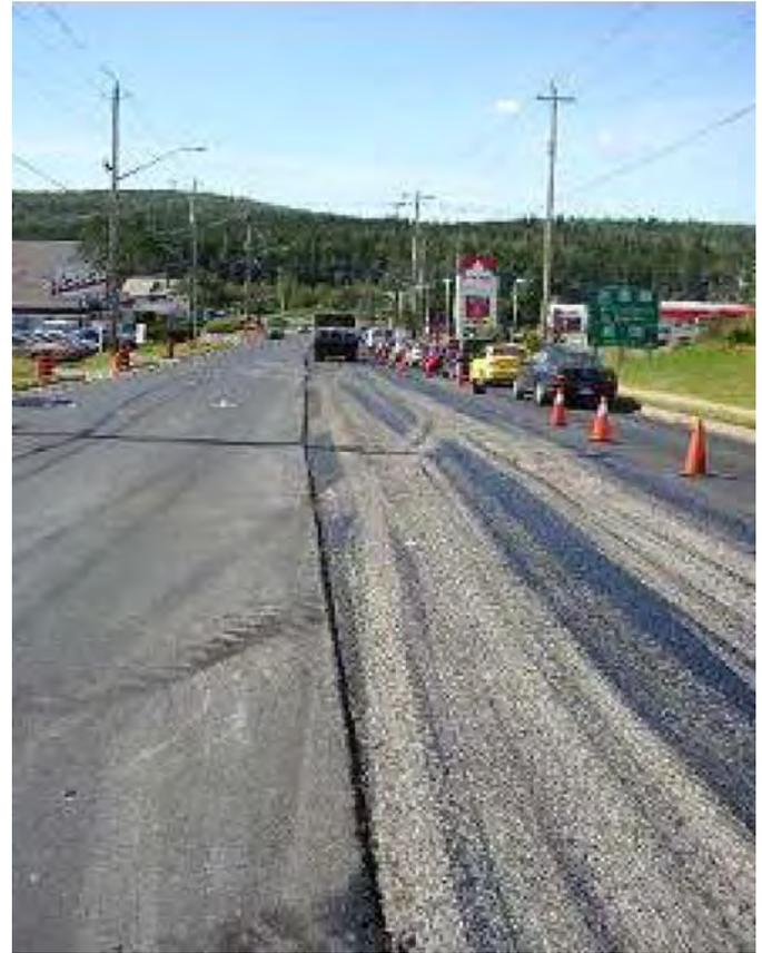
**Figure 22. Pickup of tack coat material by construction traffic.**
