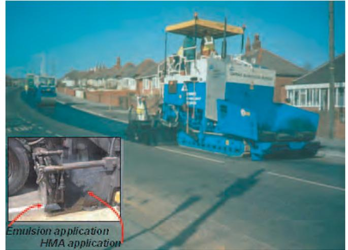
(b) Paver with tack coat tank and spray bar
