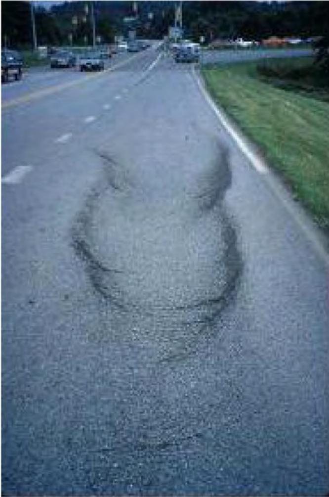
**Figure 1. Delamination type of sliding failure.**
