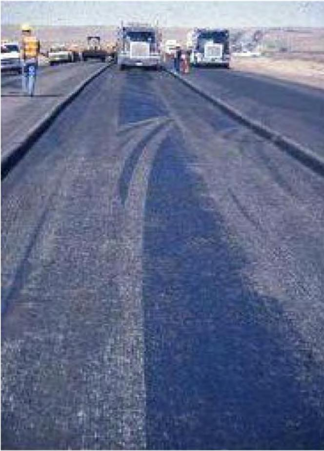
**Figure 21. Pickup of tack coat material in wheel paths by construction traffic.**
