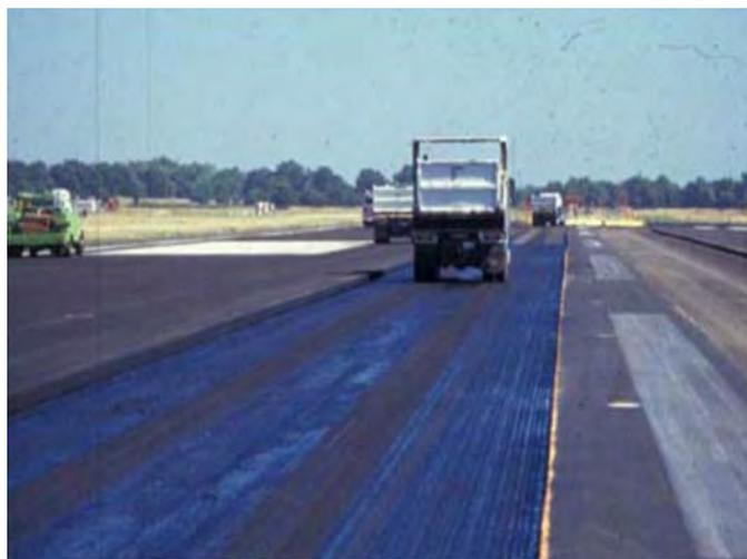
**Figure 6.** Pick-up by haul truck tires.
