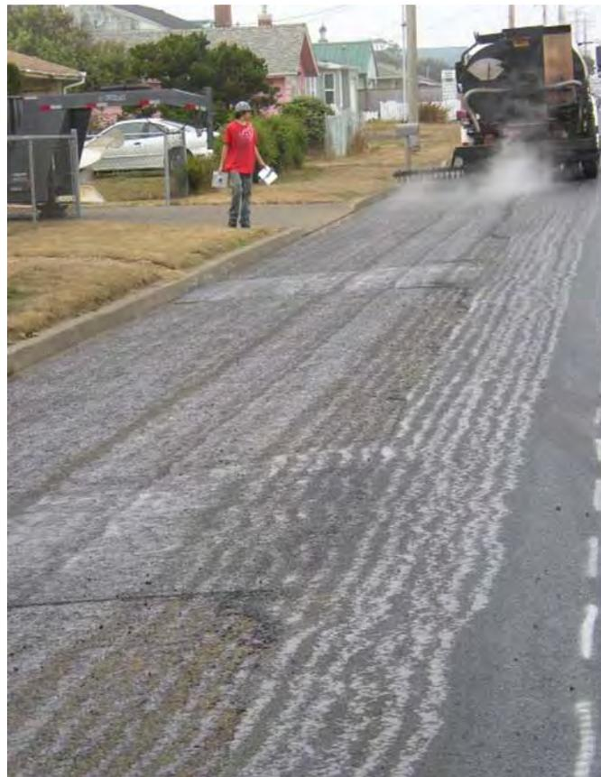
**Figure 14. Non uniform tack coat spray application.**
