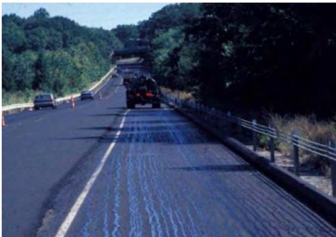
Figure 4. Non-uniform tack coat: streaks.
