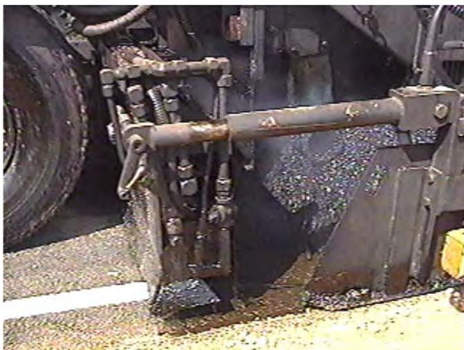
**Figure 24. Tack coat application using spray paver.**
