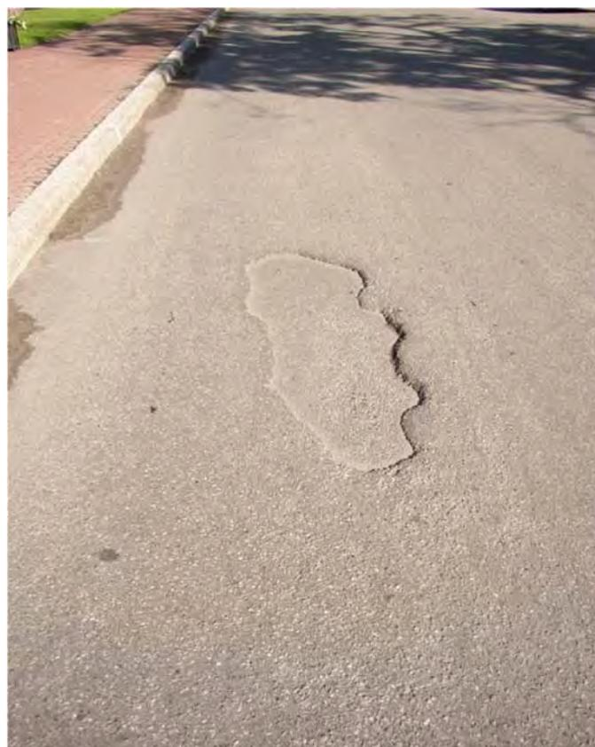
**Figure 25. Delamination failure in asphaltic concrete pavement.**
