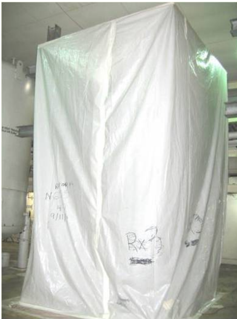
FIGURE 3-3 An example of a large item tented for monitoring at closure. SOURCE: Jeff Kiley, Chief, Quality Assurance, CMA, "CWD Closure Briefing," presentation to the committee on February 23, 2011.
