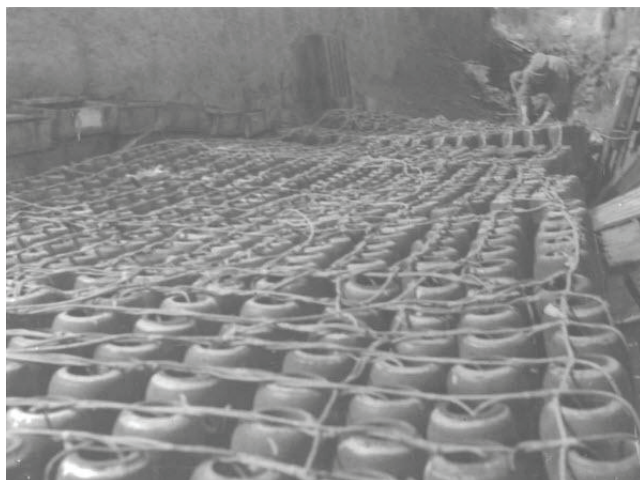
FIGURE 5-2 German Traktor rocket pit at Huntsville (now Redstone) Arsenal, Alabama (photo from 1948). SOURCE: William R. Brankowitz, Senior Chemical Engineer, Science Applications International Corporation, “The Redstone Arsenal Archival Review,” presentation to the committee on January 18, 2012.
