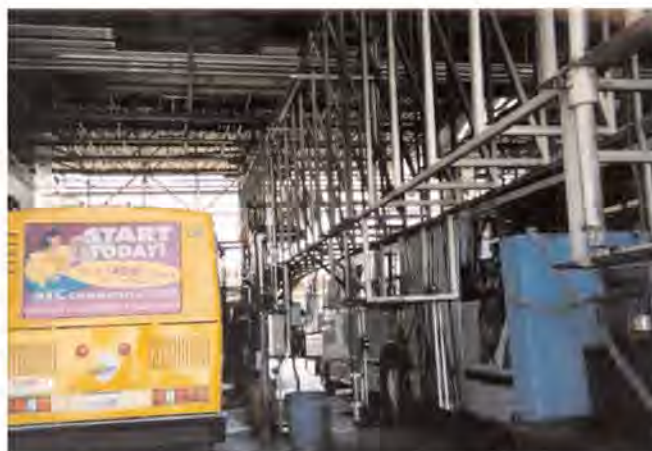
Multiple-use fuel lines surround an LNG Dallas Area Rapid Transit (DART) bus at the fueling bay.
