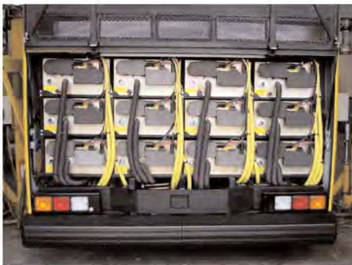
Battery compartment of a 30-ft electric transit bus.
