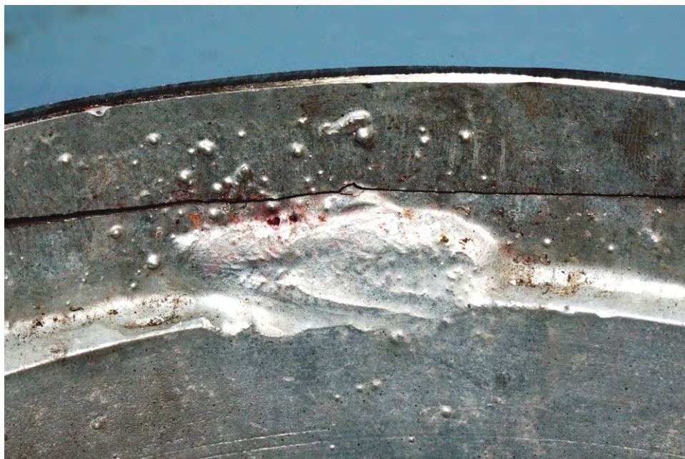
Figure 44 Fatigue cracking in arm of specimen III-5 from tack weld between the backing ring and the tube wall
