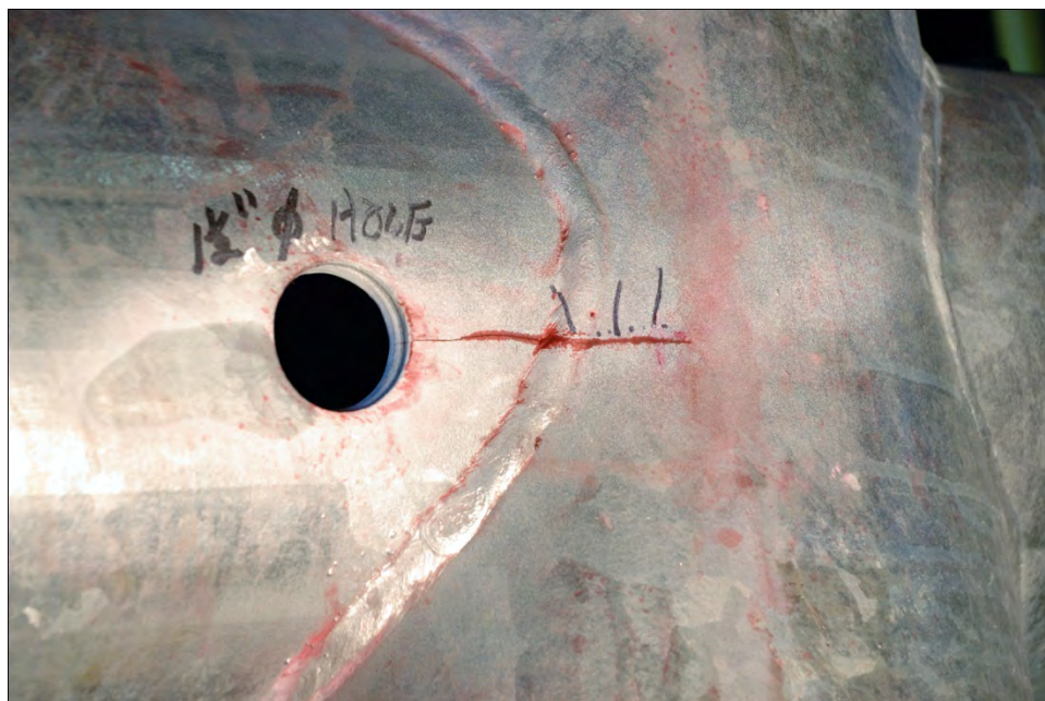
Figure 50 Fatigue cracking in specimen VI-1 from weld root arrested by hole drilling in the arm sleeve
