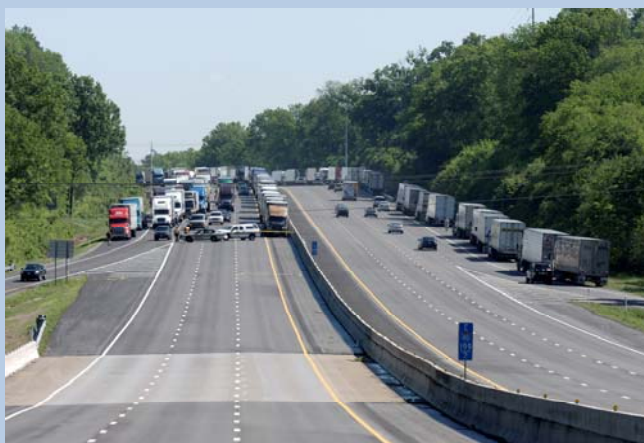
Traffic on I-40, a major east–west corridor across the United States, halted in West Nashville, Tennessee, due to flood waters after heavy rainfall in May 2010.
