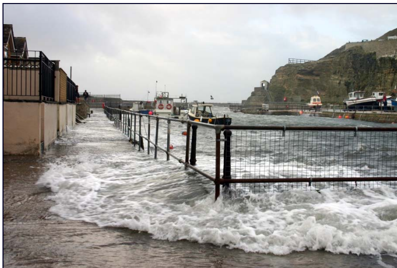
Harbor floods during heavy storm, Cornwall, United Kingdom.
