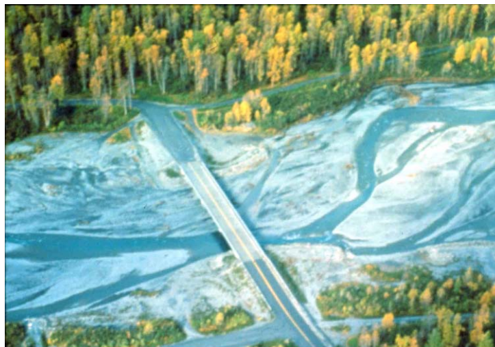
Figure 5-4. Bridge crossing of a braided channel.
