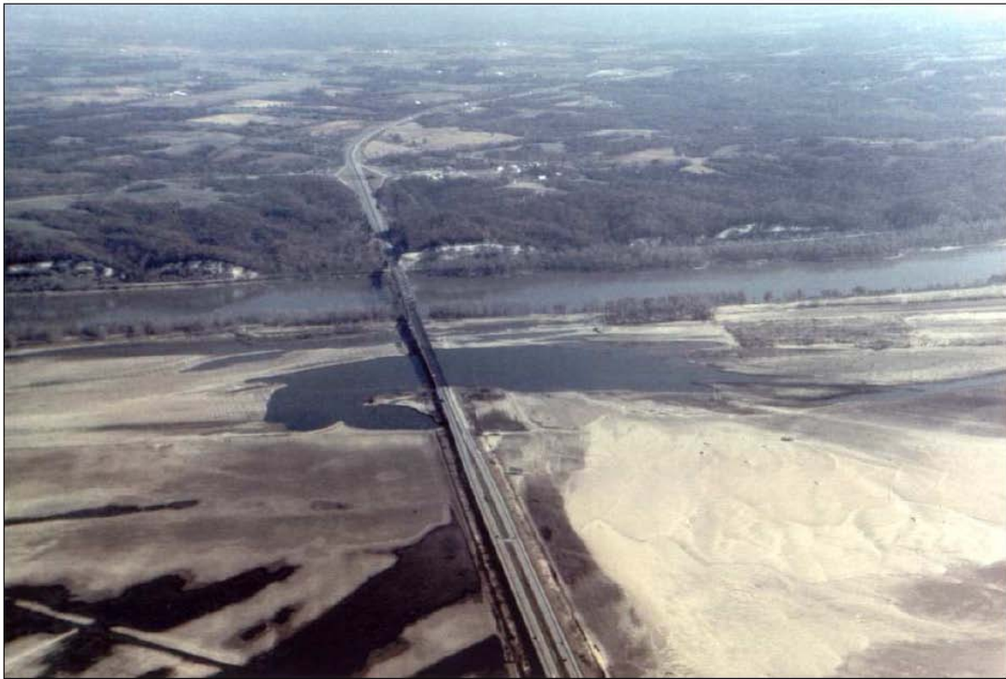
Figure 1-4. Scour at I-70 bridge over Missouri River from 1993 flood. Flow was from left to right. (Photo from Parola et al. 1998).
