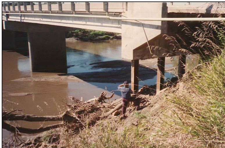
Figure 3-1. A common situation of abutment failure; scour has led to failure and partial washout of the earthfill spill-slope at this abutment. A basic question arises as to how abutment design should take scour into account.
