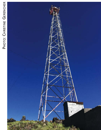
Air traffic control technology always has adapted to the needs of the region served. Developed in the 1920s and 1930s, the lighted airway beacon system has been phased out in most of the United States, but “OriginalGen” remains in service in the remote, mountainous regions of Montana.
