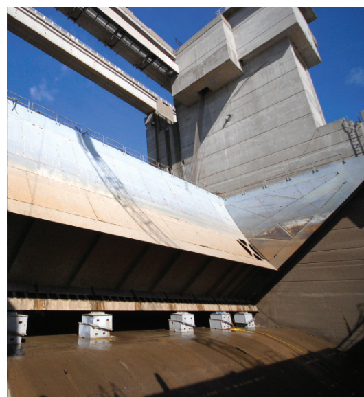
PHOTO: GEORGE STRONGMAN, U.S. ARMY CORPS OF ENGINEERS
