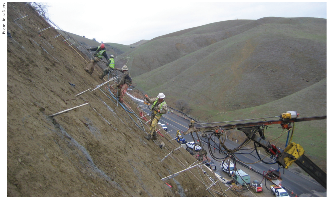
Installation of soil nails and wire mesh in California.
