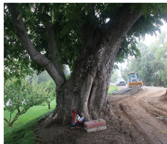
An aged walnut tree on a levee along the Sacramento River in California. A 2009 Corps study examined the effects of the root systems of trees and vegetation on levees and slurry walls.
