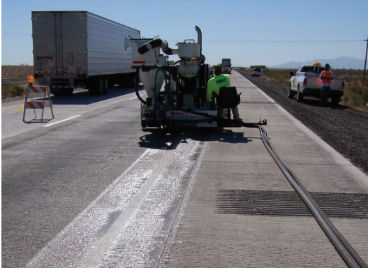
Concrete slab grinding at an Arizona test site. Surface smoothness is one of the protocols developed for the pooled-fund study.
