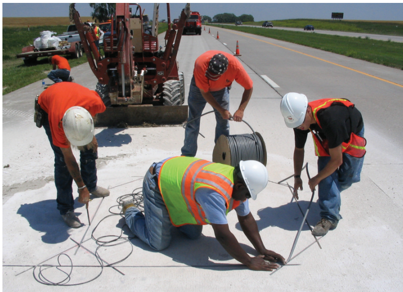
Phase II contractors install an inductive loop at a Kansas test site.
