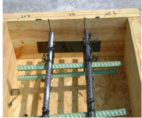
(b) Plate used to ensure proper layer separation
