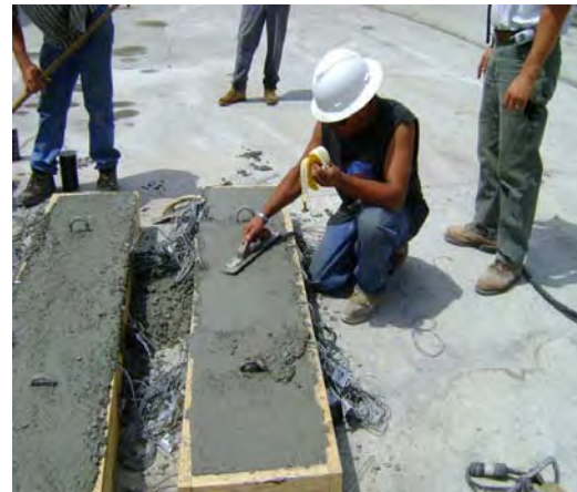
(f) Concrete finishing
