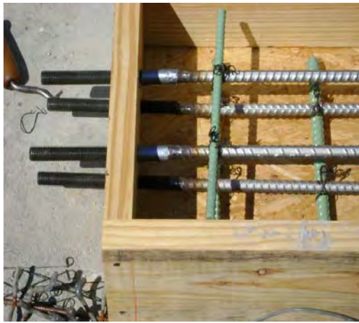
(c) Threaded rods extending through the form
