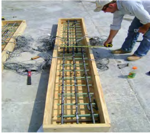
(a) Reinforcement in the forms
