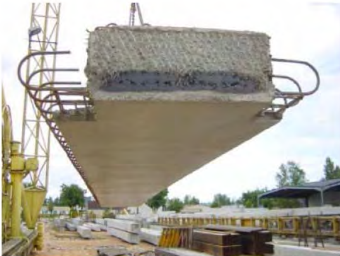
Figure 2.1.1: Photograph of precast section used in Poutre Dalle System (Hagen, 2005)
