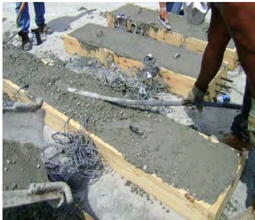
(e) Vibrator use in the joint zone
