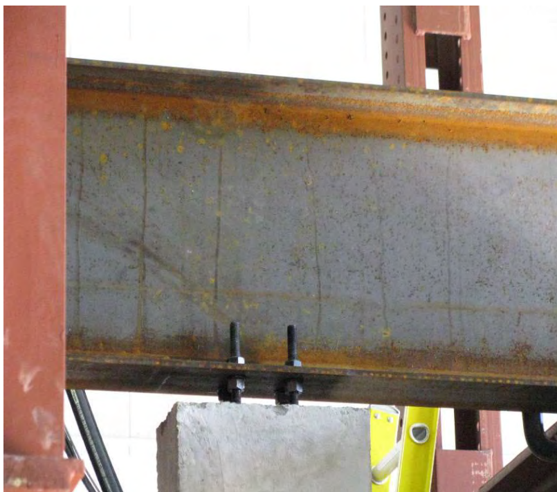
Figure 9.1.13: Photo of the top connection detail
