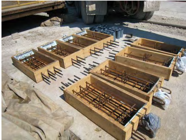
(a) Before pouring
