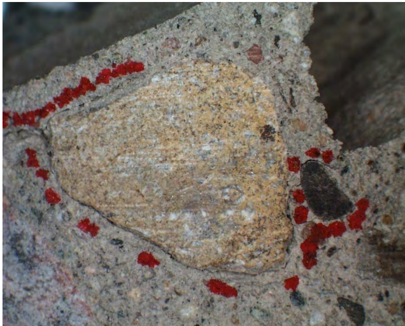
Figure G2: Identified crack marked on core specimen using red ink
