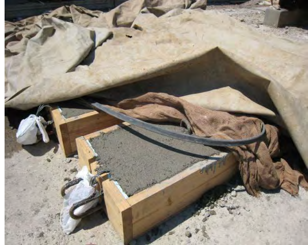
(b) After pouring and curing
