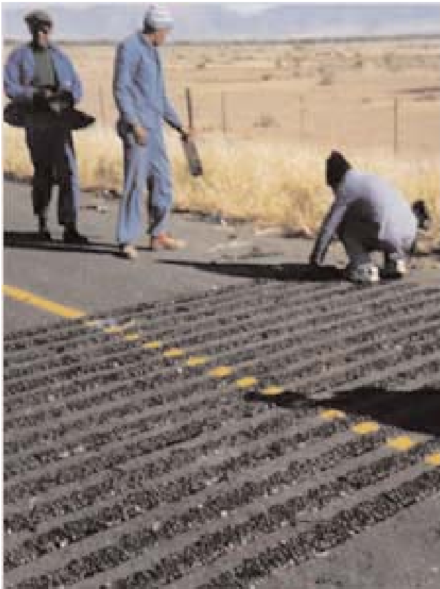
FIGURE 16 Rumble strips. Source: A.J. Broom Road Products.
