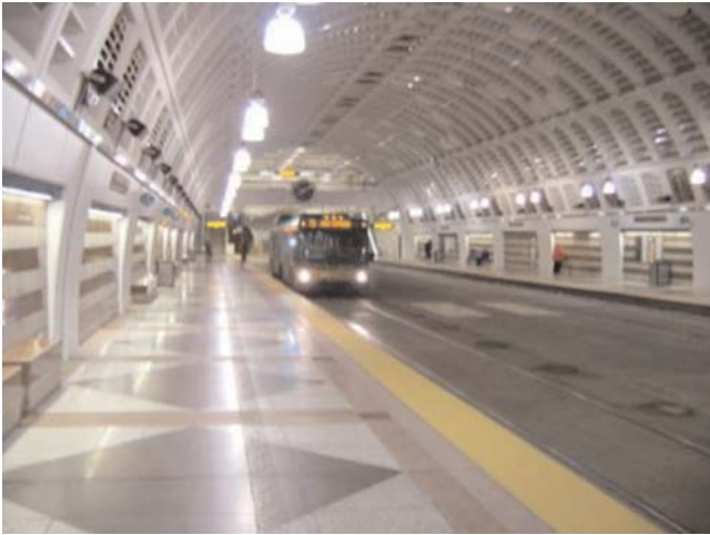
FIGURE 6 Tunnels that accommodate bus stops (Seattle).
