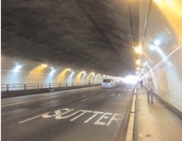
FIGURE 5 Tunnel with pedestrian walkways all along the tunnel for pedestrian crossings (San Francisco).
