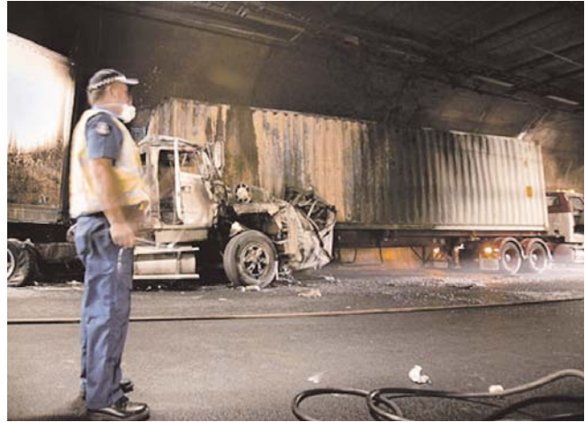
FIGURE 4 Burnley Tunnel (Australia) after fire.
