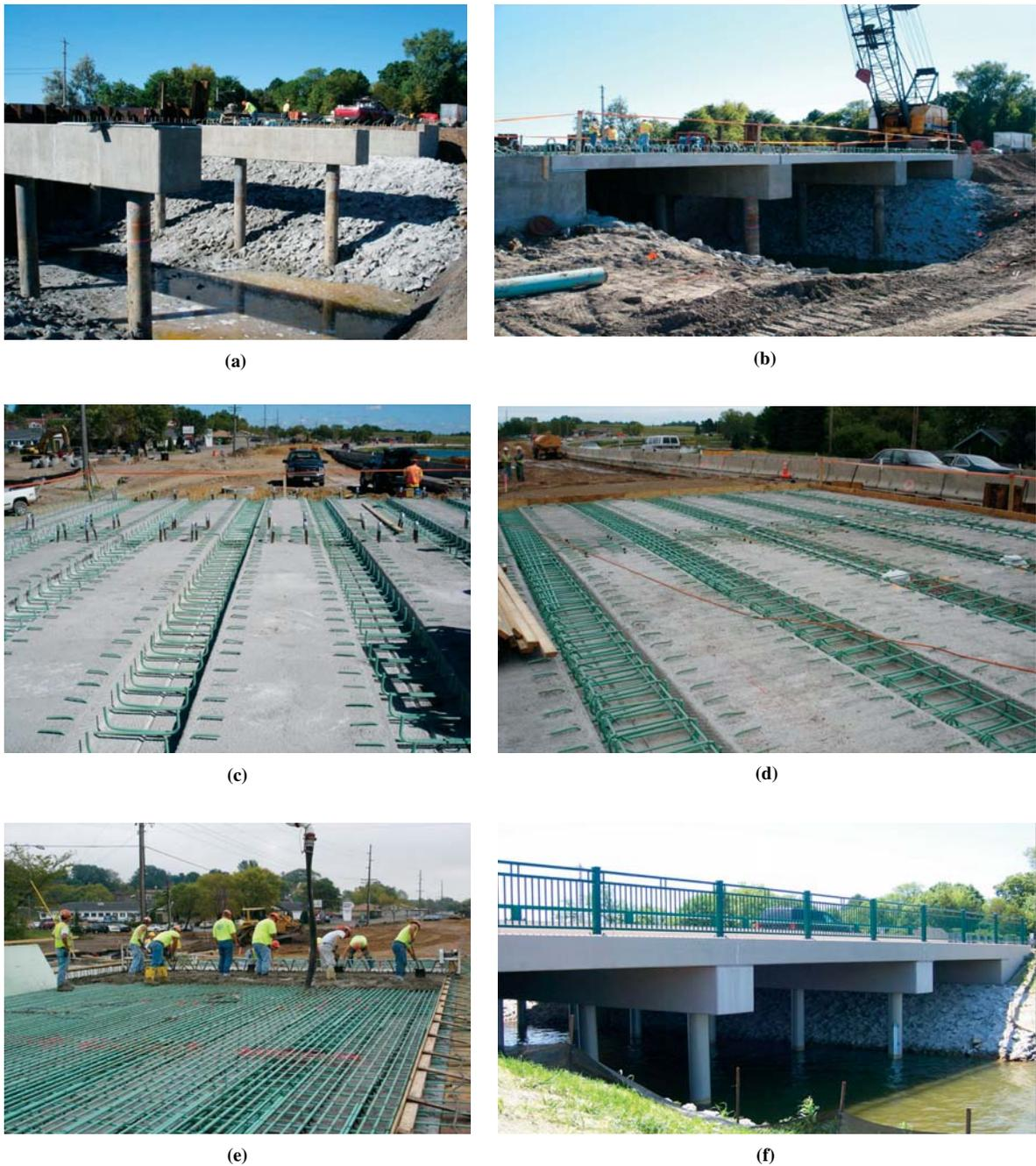
**Figure 1** Sequence of construction of a PCSSS: (a) precast pier caps in place, (b) Inverted T-sections in place (elevation view), (c) Inverted T-sections in place (plan view), (d) drop-in cage placed between precast webs for potential crack control, (e) deck reinforcement in place, and (f) finished structure.
