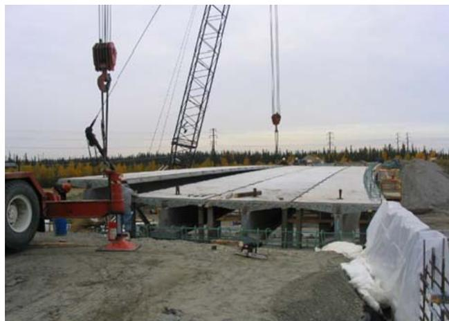
**Figure 15** A DBT concrete bridge being constructed.
